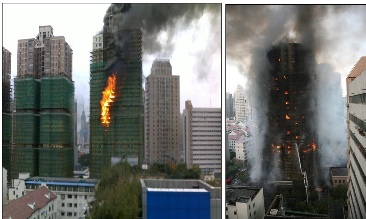
Figures 1 and 2 – The high-rise apartment building fire at Jiaozhou Road, Shanghai, China 2010
