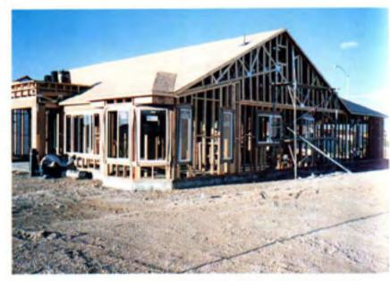
Modern timber frame 'stick' construction is responsible for excessively rapid fire escalation and early collapse – see Chapter 8.
