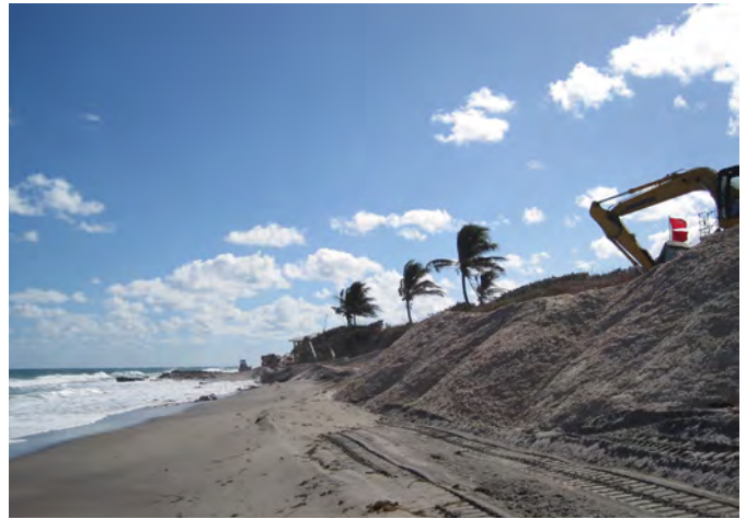
Dune restoration in progress ©Palm Beach County Environmental Resource Management
