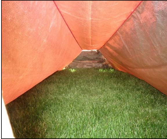
Figure 7: Single tarp interior using dual roof support cords and raised end wall
