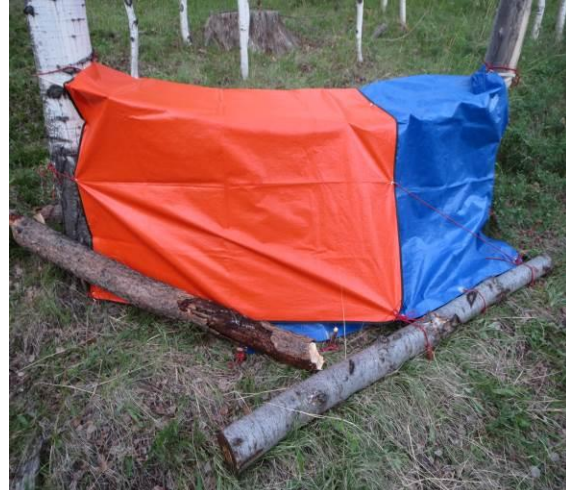
Figure 14: Completed shelter; contrasting tarps show “shingle” concept; R log is entry closure and anchors both tarps
