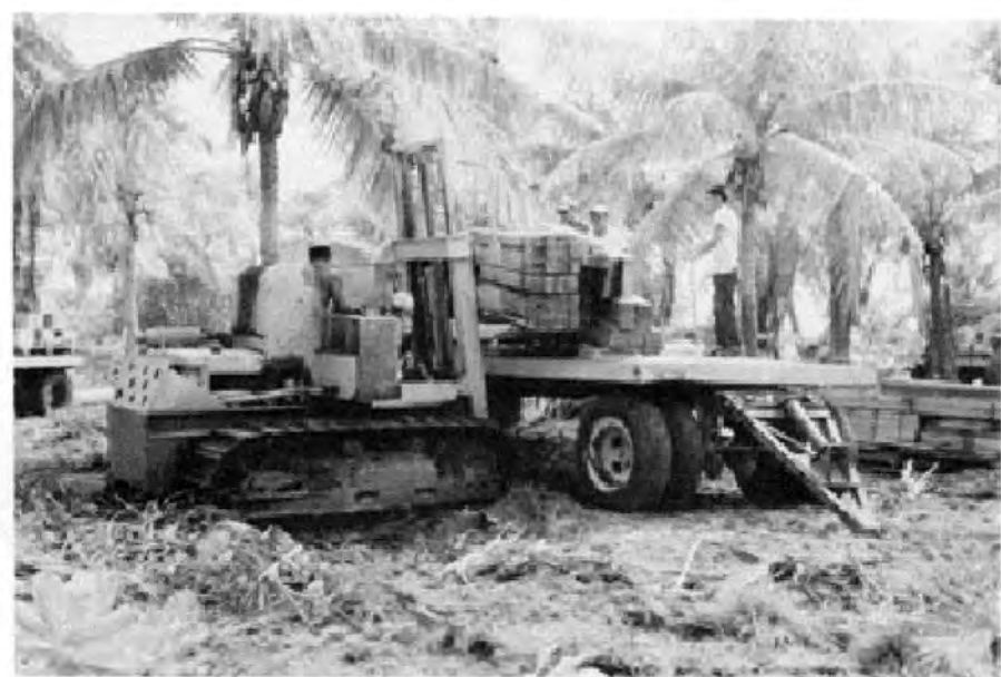
FIGURE 1-39. TRANSPORTING CONSTRUCTION MATERIALS ON ENEWETAK.
