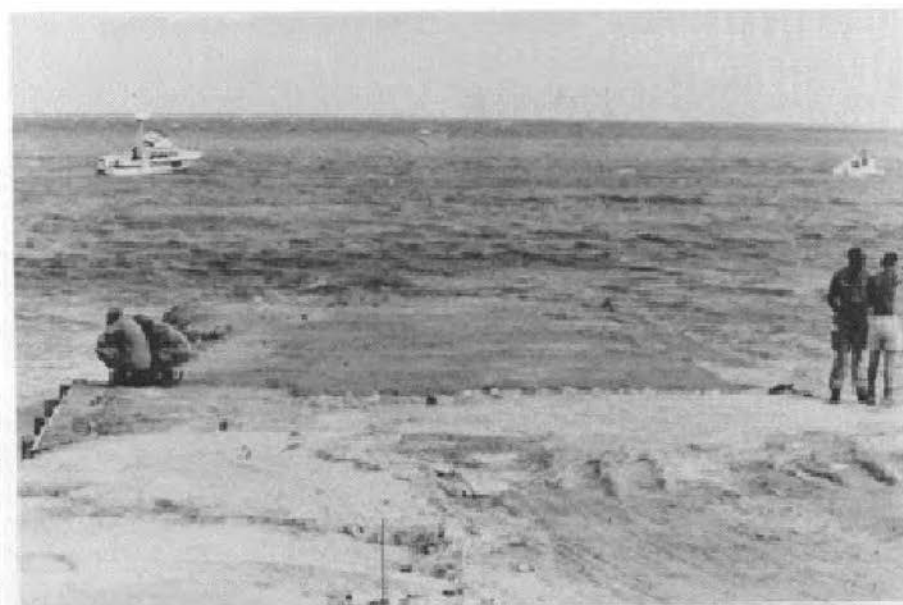
FIGURE 10-30. ENEWETAK BARGE JETTY.
