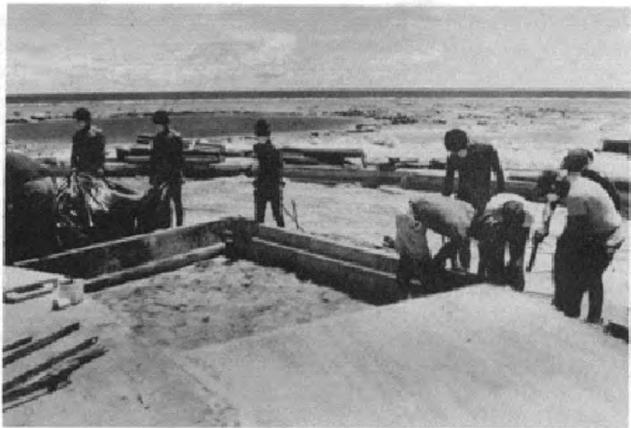
FIGURE 8-45. WOODEN CAP FORMS WITH TAPERED KEY.
