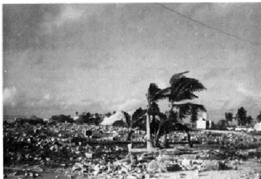
FIGURE 4-15. DEBRIS FROM TROPICAL STORM NADINE.
