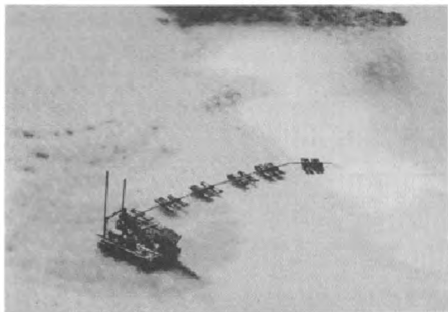
FIGURE 7-41. AOMON SANDBAR DREDGING.
