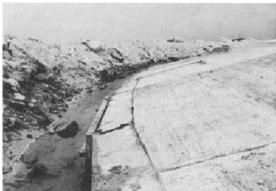
FIGURE 8-43. KEYWALL EXPANSION JOINT.
