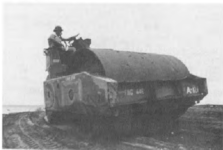
FIGURE 8-33. COMPACTING SOIL-CEMENT MIXTURE.
