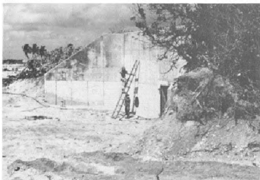
FIGURE 5-25. BUNKER SAND-BLASTING OPERATION.
