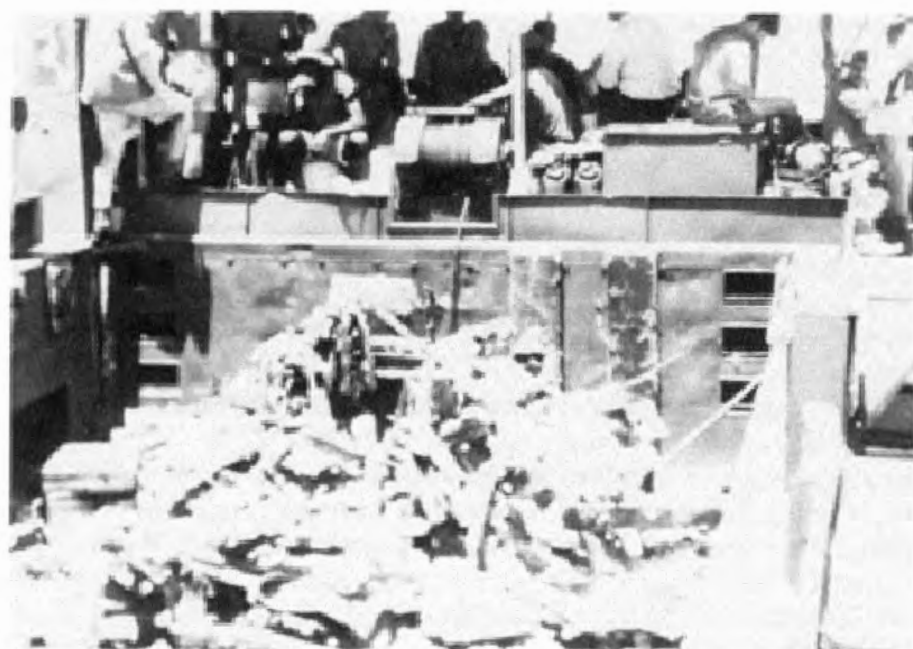
FIGURE 5-7. DEBRIS LOADING, LARC-LX.
