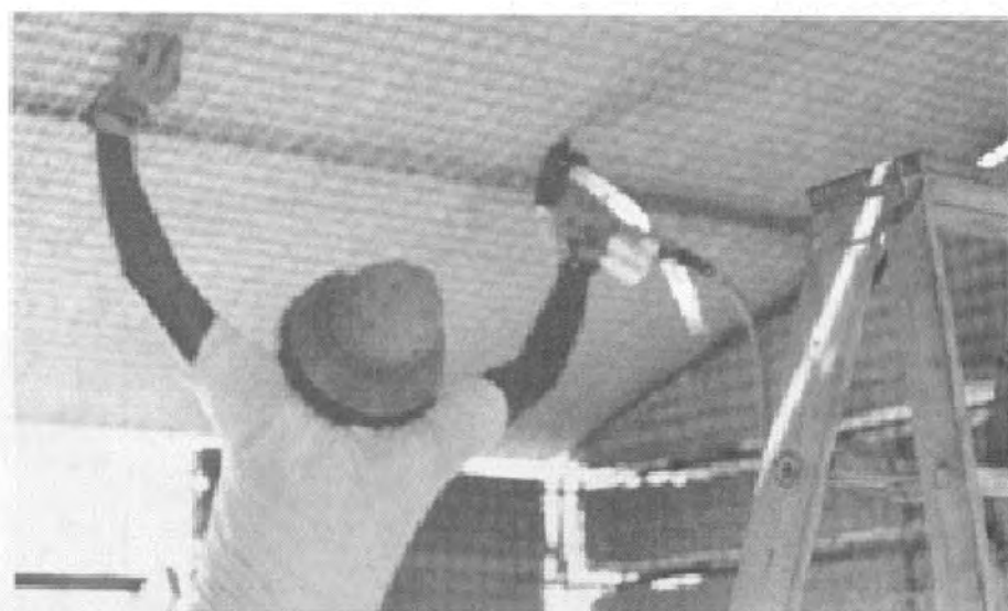
FIGURE 10-14. JOINING CEILING PANELS WITH AIR-ACTUATED CLAMPING DEVICE.
