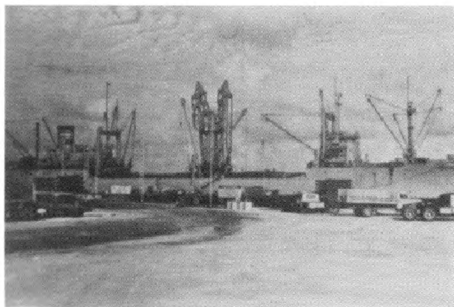
FIGURE 1-38. UNLOADING MATERIAL AND EQUIPMENT AT MEDREN PIER.
