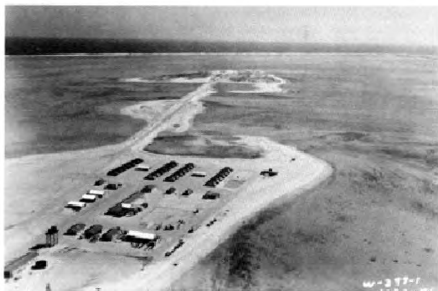
FIGURE 1-44. CONSTRUCTION CAMP ON LIDILBUT (GENE) ISLAND.
