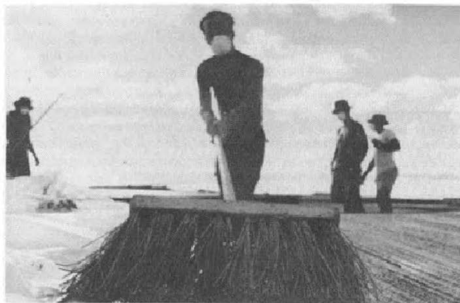
FIGURE 8-48. BROOM-FINISHING A CAP SECTION.
