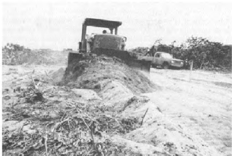
FIGURE 6-4. SOIL REMOVAL USING D8K DOZER.
