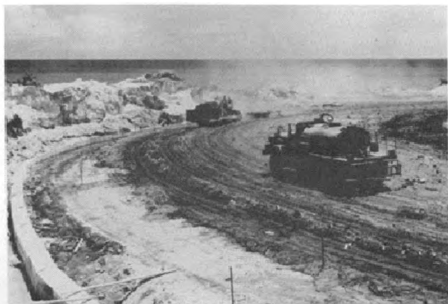
FIGURE 8-32. SPRINKLING SOIL-CEMENT MIXTURE.
