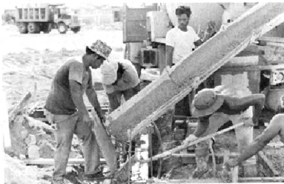
FIGURE 10-12. PLACING CONCRETE FOR HOUSE FOOTINGS.
