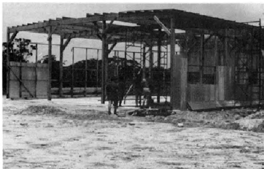
FIGURE 3-8. LOJWA BUILDING CONSTRUCTION.
