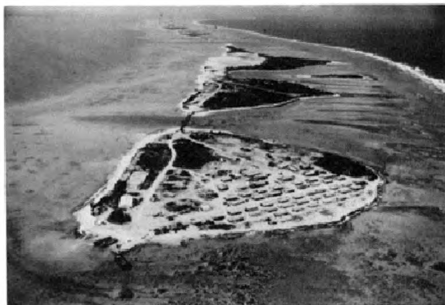
FIGURE 3-20. COMPLETED LOJWA BASE CAMP.
