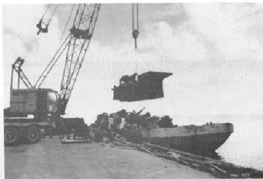
FIGURE 5-16. DUMP BED OFFLOADING.
