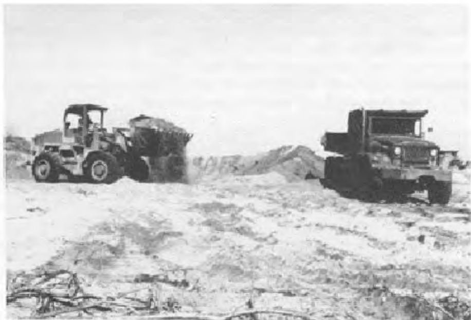
FIGURE 6-9. CONTAMINATED SOIL MOVEMENT.
