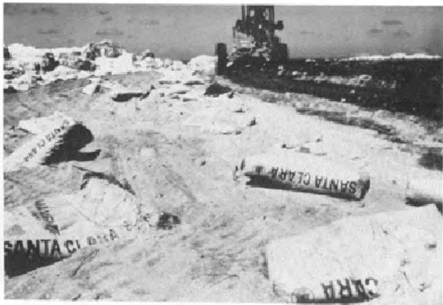
FIGURE 8-30. CEMENT BAGS PLACED FOR SOIL-CEMENT MIX.
