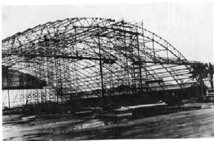
FIGURE 1-41. ERECTION OF AIRCRAFT HANGAR.
