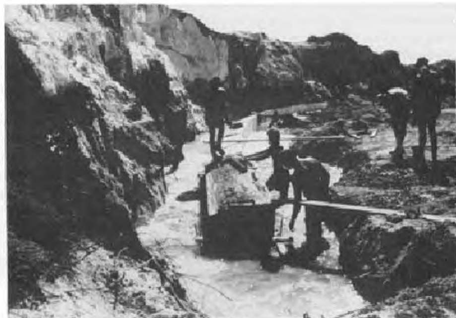
FIGURE 8-26. BUILDING THE KEYWALL.
