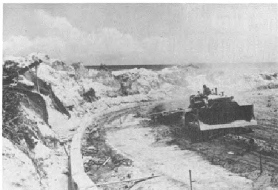
FIGURE 8-31. MIXING SOIL AND CEMENT WITH DISC HARROW.
