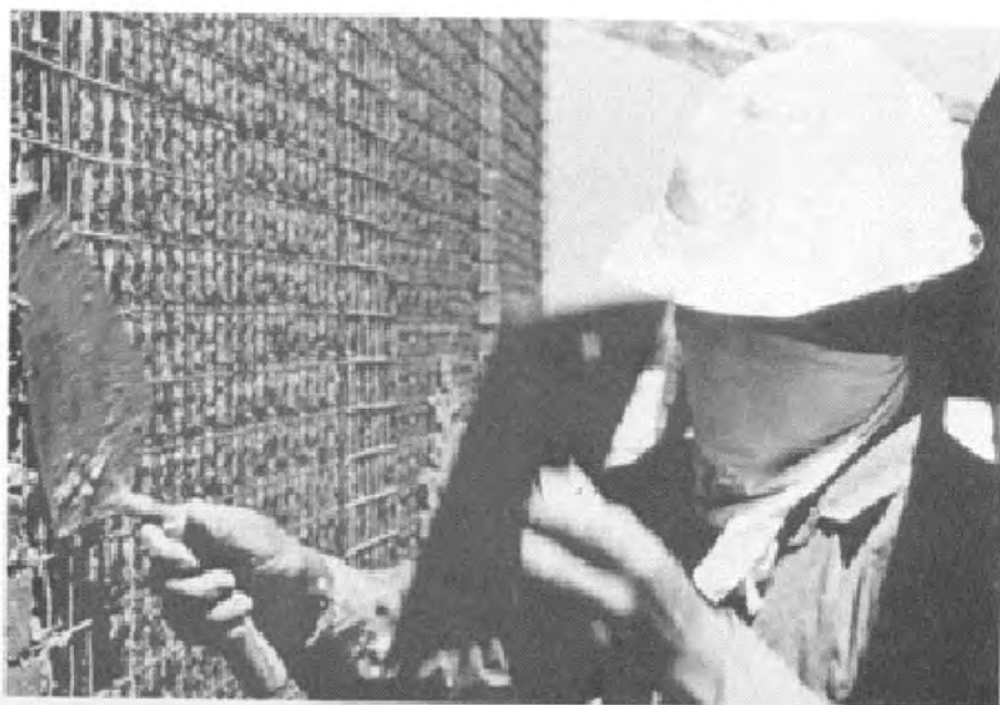
FIGURE 10-16. APPLYING CEMENT PLASTER.
