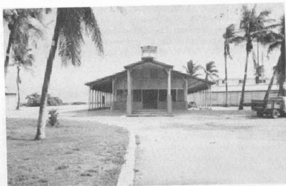
FIGURE 10-25. CHURCH ON ENEWETAK ISLAND.
