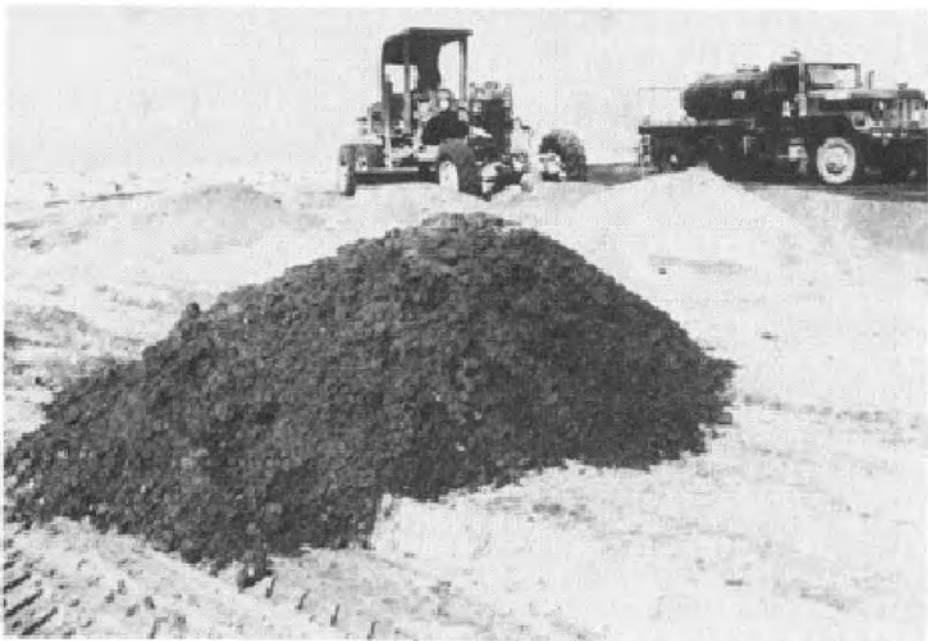
FIGURE 8-29. SPREADING SOIL WITH A GRADER.
