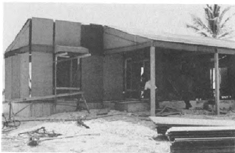
FIGURE 10-15. HOUSE NEARING COMPLETION WITH W-PANELING INSTALLED.
