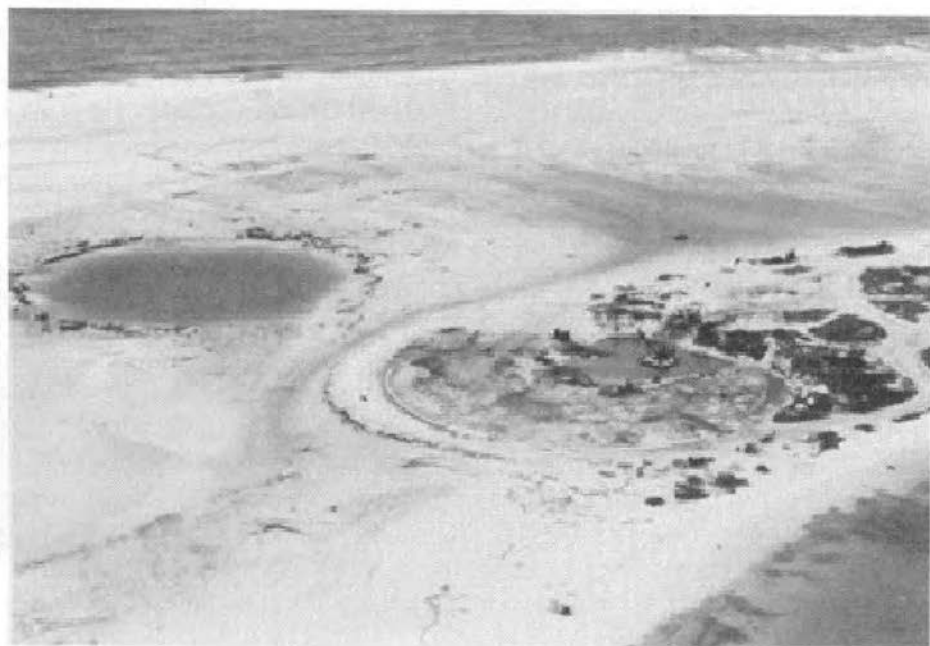
FIGURE 8-25. TREMIE OPERATIONS NEARING COMPLETION.
