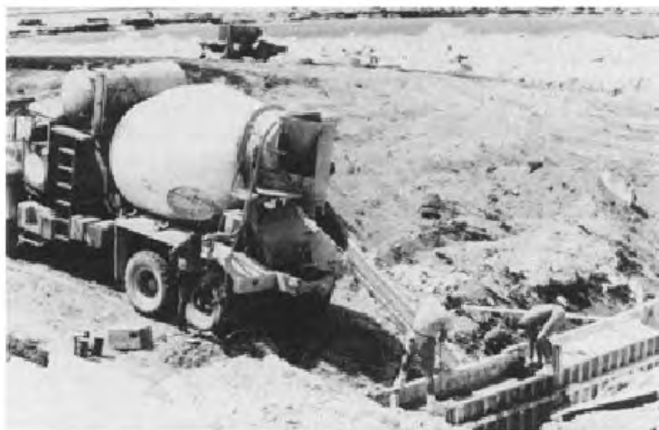
FIGURE 8-27. PLACING CEMENT IN KEYWALL FORMS.
