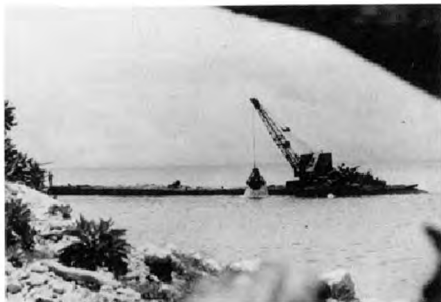
FIGURE 5-9. FLOATING PLATFORM DEBRIS REMOVAL.
