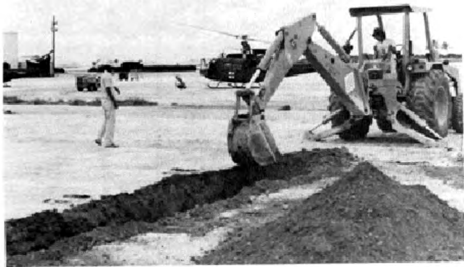
FIGURE 10-11. STARTING HOUSE CONSTRUCTION.
