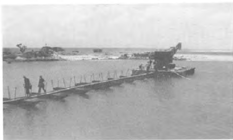
FIGURE 8-22. TREMIE BARGE AND CRANE.
