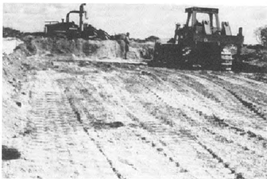
FIGURE 6-6. BACKBLADING OPERATION.
