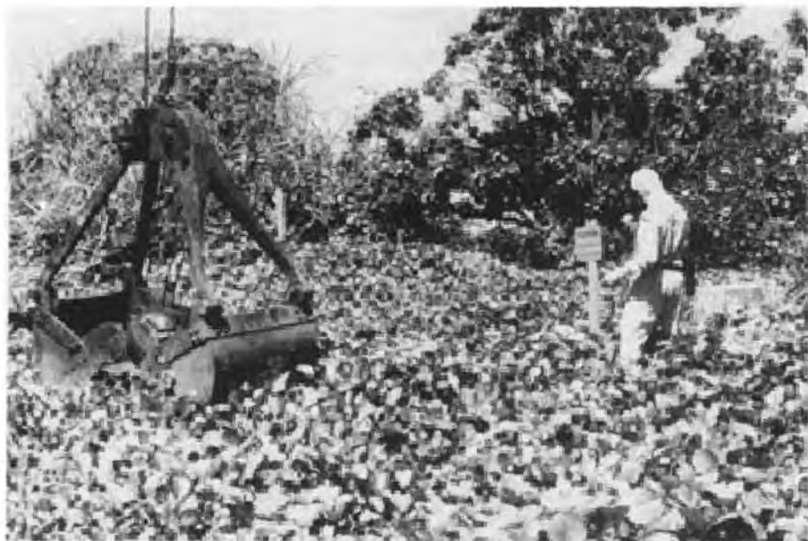
FIGURE 7-34. ADMON CRYPT INITIAL EXCAVATIONS.
