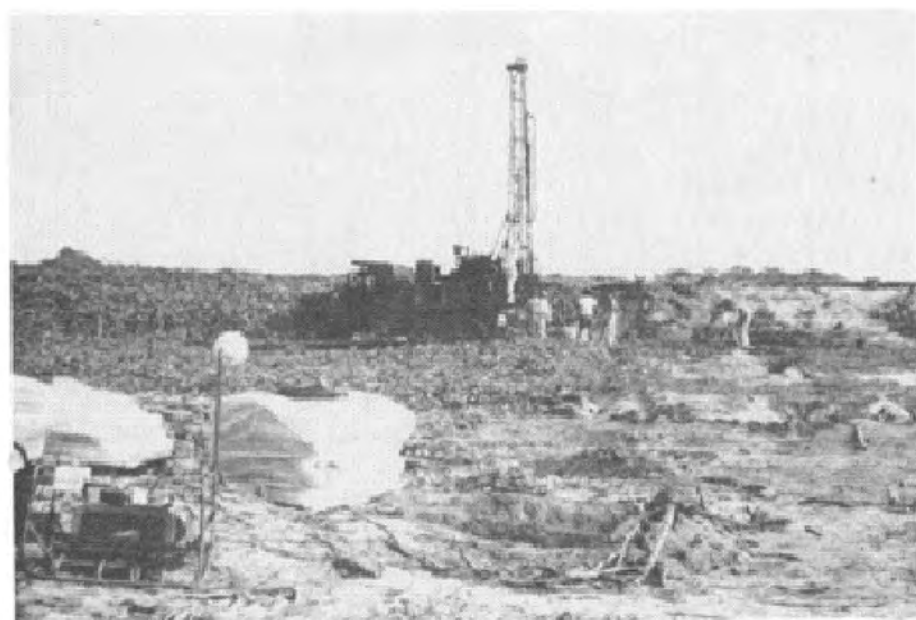
FIGURE 7-30. DEEP DRILL SAMPLING.
