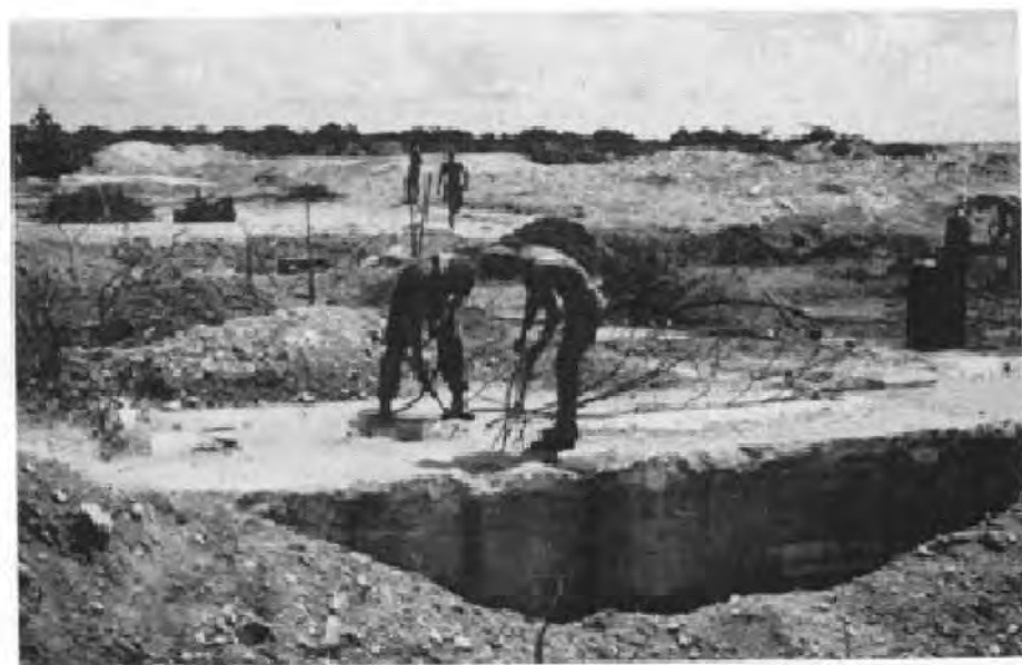
FIGURE 5-24. ENJEBI HILTON AFTER DEMOLITION.
