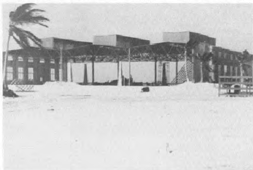
FIGURE 1-46. HANGARS CONSTRUCTED TO STUDY BLAST EFFECTS, ENJEBI.
