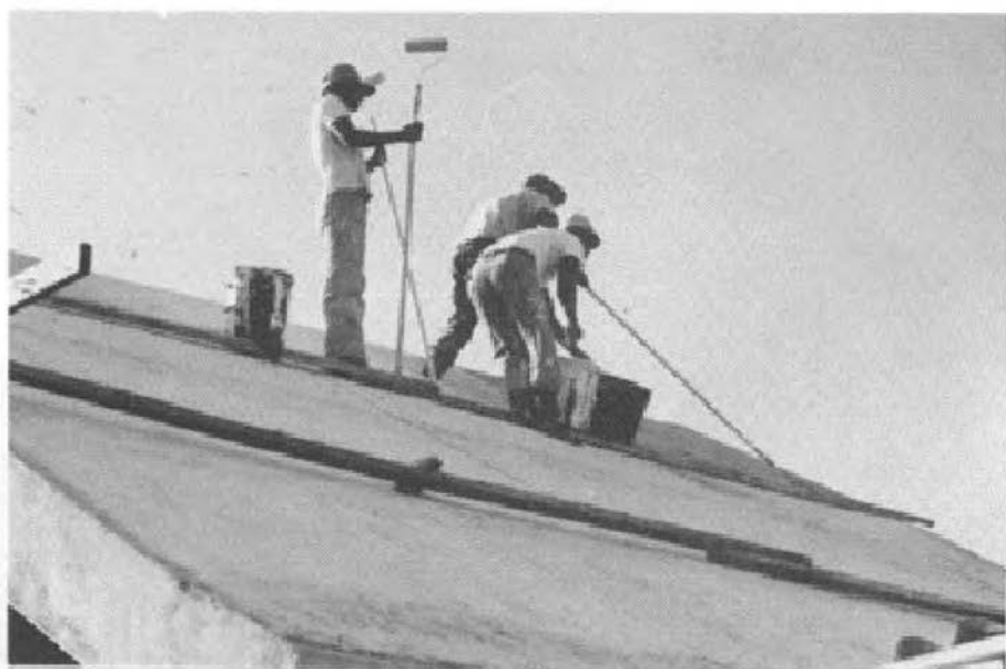
FIGURE 10-18. PAINTING THE ROOF.
