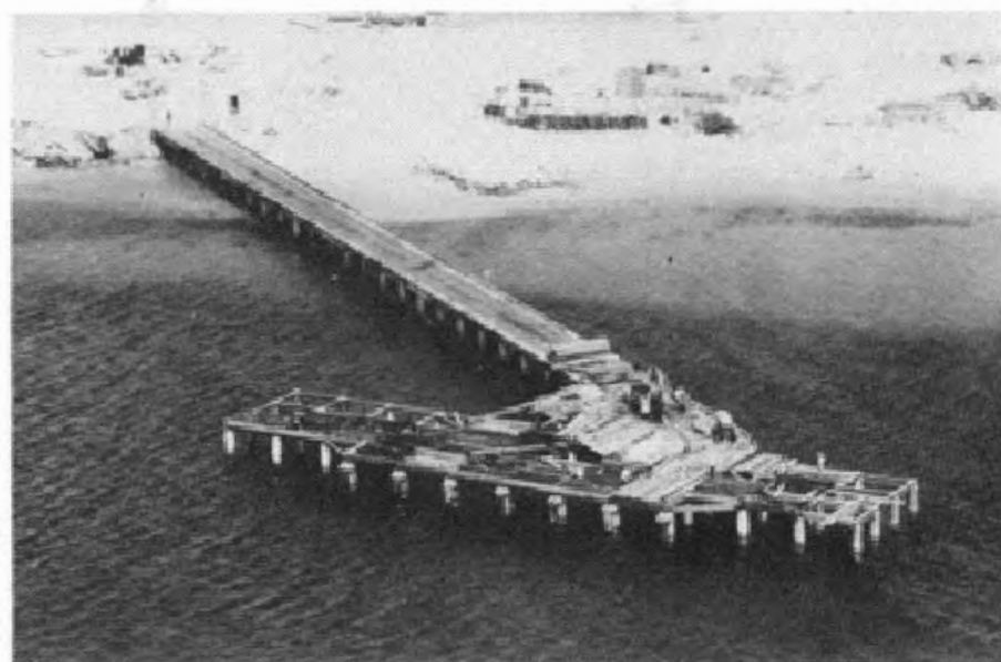
FIGURE 10-27. DEEPWATER PIER ON MEDREN, UNDER CONSTRUCTION.
