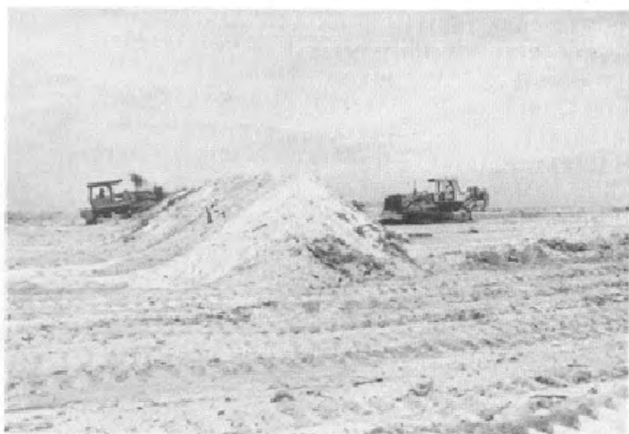
FIGURE 6-7. SOIL WINDROWING.
