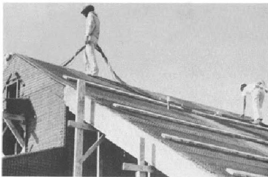
FIGURE 10-17. PNEUMATIC APPLICATION OF CEMENT PLASTER TO A ROOF.
