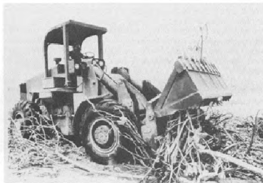
FIGURE 6-5. BRUSH REMOVAL USING FRONT LOADER.
