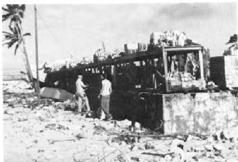
FIGURE 7-19. TYPHOON ALICE DAMAGE, DRY STORES.
