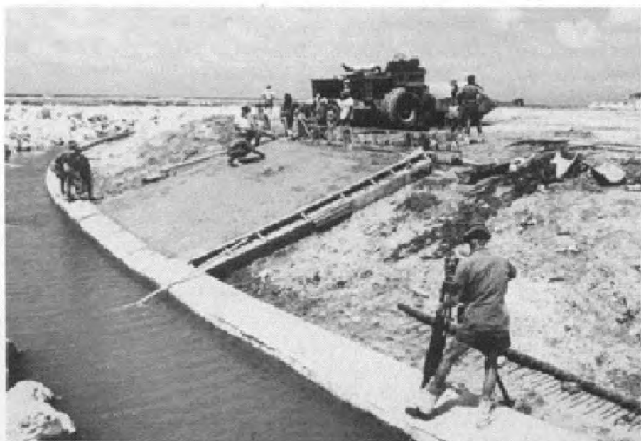
FIGURE 8-44. SIDE VIEW OF FORMS.
