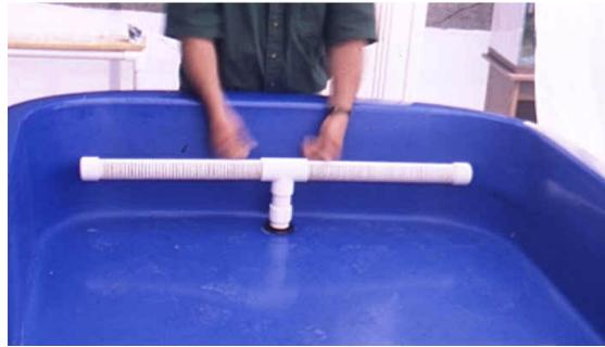
**Figure 5: Pressing Drain Header into Drain Bulkhead Assembly**
