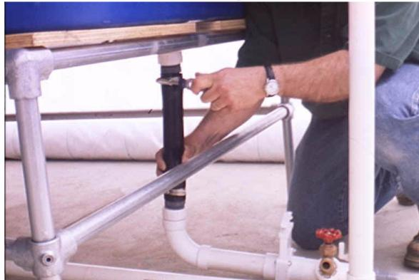
**Figure 4: Installing Valve Assembly**
