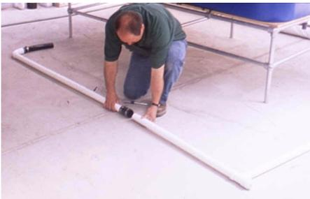
**Figure 6: Assemble Return Line parts on the floor for flatness**
