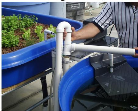
**Figure 9: Push Return Flow and Skimmer pipes down onto top of Airlift pipe**
