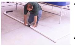
Figure 6: Assemble Return Line parts on the floor for flatness
