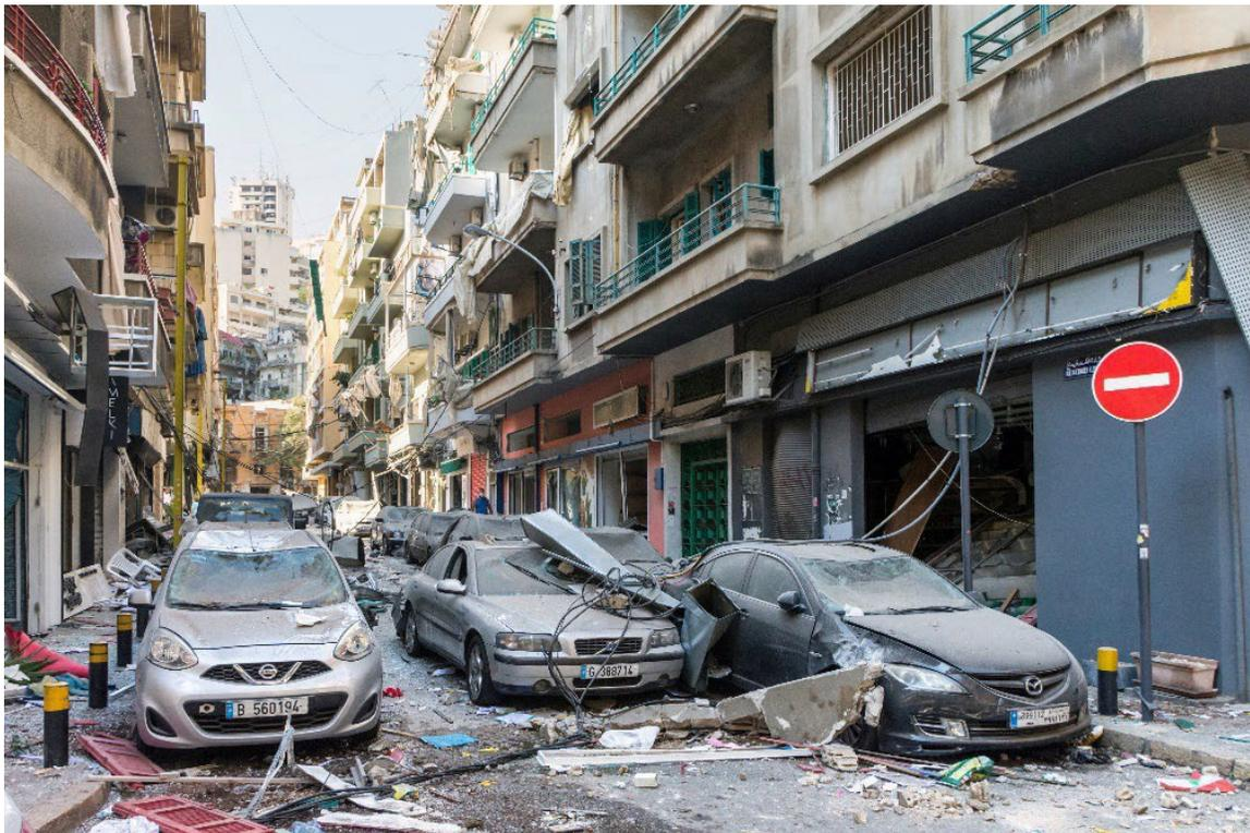
**Figure 7. Example of Anticipated Impacts In Light Damage Zone.<sup>24</sup>**
