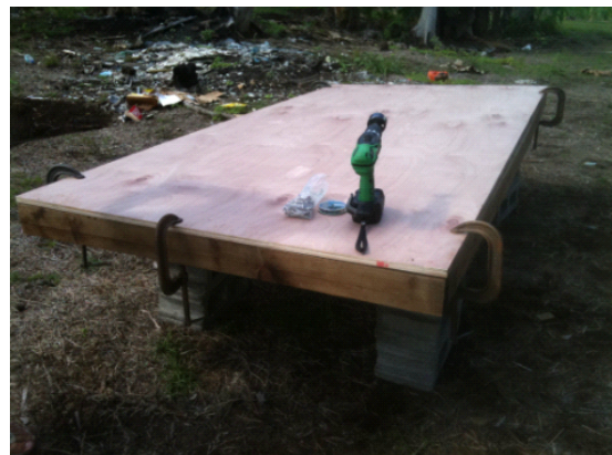
Figure 3. Bottom of tray ready to be screwed to sides.
