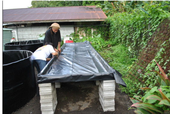
Figure 4. Attaching liner to the tray.
