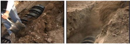
Figure 18. Once the chambers are placed backfill the sides of the chamber prior to backfilling the trench. Failure to do this my result the chambers collapsing.
