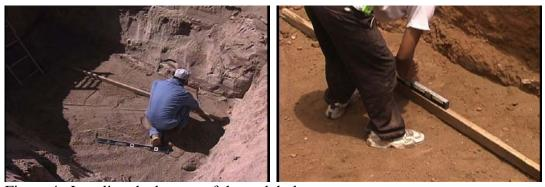
Figure 4. Leveling the bottom of the tank hole.
