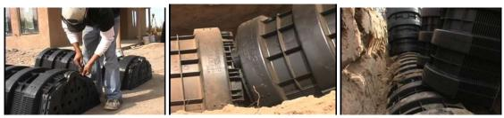
Figure 17. Screw in the end plate and then place the chambers in the trench in sequence.
