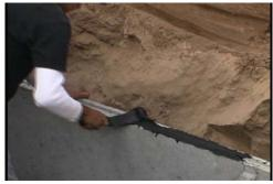
Figure 5. You should be present when your septic tank is installed. If the tank is a split tank make sure the entire joint is filled with mastic prior to tank assembly.
