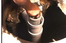
Figure 6. An outlet filter or bioscreen in the septic tank is required.
