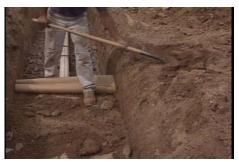
Figure 15. Backfilling the gravel and pipe system.
