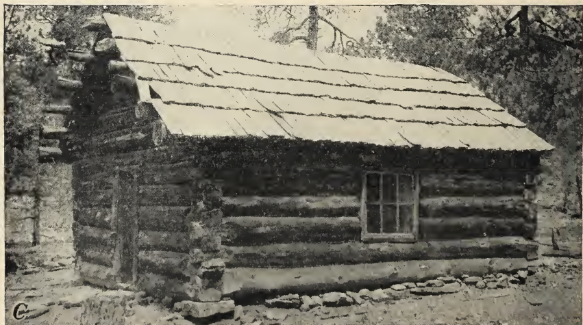
FIGURE 35.—Early types of log structures built by the U. S. Forest Service in the West. A , Ranger station, Gallatin National Forest, Mont.; B , ranger's dwelling, Nezperce National Forest, Idaho; C , log cabin in Arizona.
