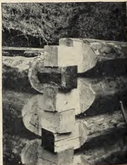
FIGURE 6.—Marking and framing the dovetail, or box, corner.
