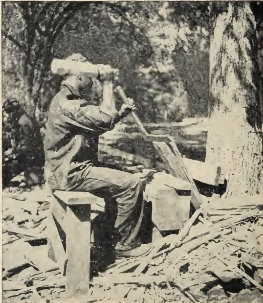
FIGURE 20.—Splitting shakes with the froe.
