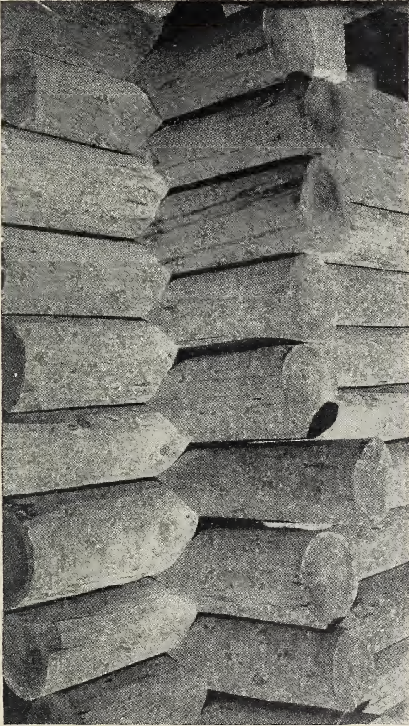
FIGURE 2.—The round-notch or saddle corner. This is an unusually fine example of scribing and fitting logs together. The square-cut logs have yet to be dressed and shaped with the ax to give them a pleasing appearance.
