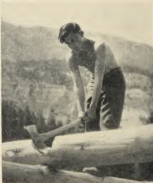
FIGURE 5.—Chopping the notch in a saddle corner.
