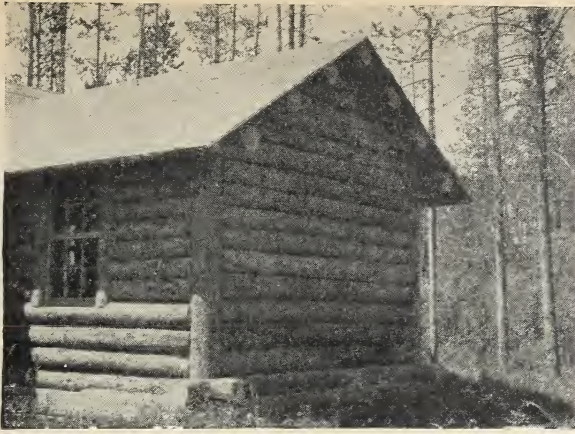
UPRIGHT OR GROOVE AND TENON CORNER
