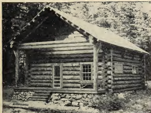
LOG BRACKETS UNDER EAVE SHAKES SUPPORT INCREASED OVERHANG
