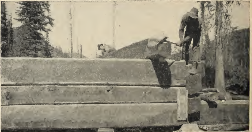
FIGURE 20.—Framing hewed timbers.
