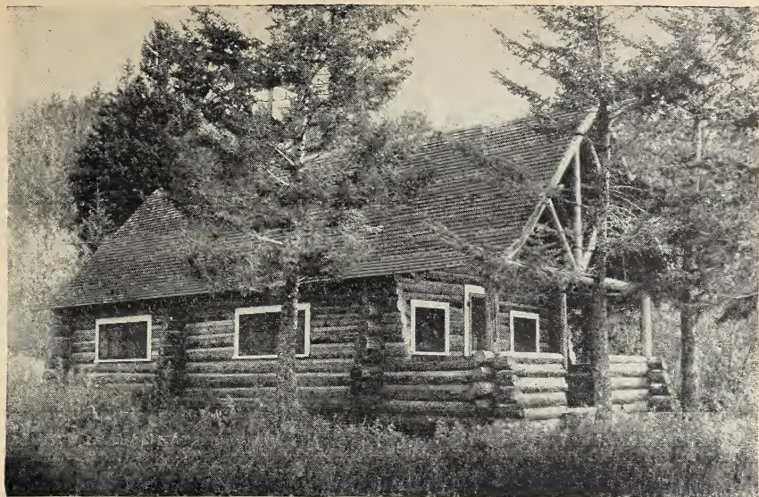
FIGURE 32.—A useful type of modern log dwelling—ranger station, Gallatin National Forest, Mont.
