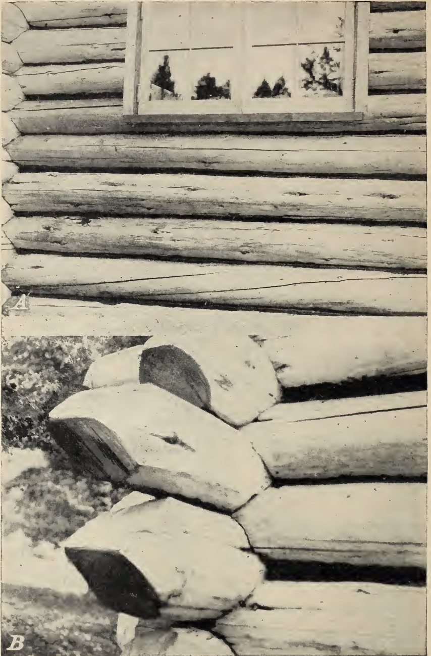
FIGURE 24.—Examples of tight joints well calked. A , Interior calking; B , exterior calking.
