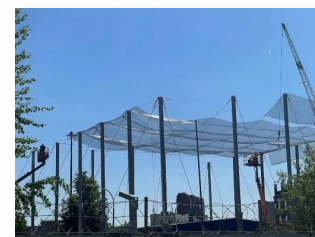
Top: Netting used to protect fans from projectiles can be repurposed to disrupt sUAS flight and observation. Bottom: Anti-drone netting installed to protect critical infrastructure from overhead threats..
