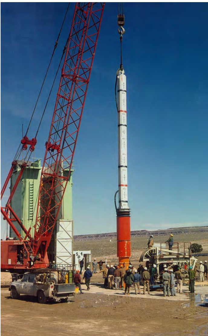
Handley was conducted on March 26, 1970, in hole U20m in the northwestern part of the NNSS. The test yield was more than 1 Mt, one of the largest detonations conducted at the NNSS. The downhole emplacement of the Handley device and diagnostics rack is shown above.
