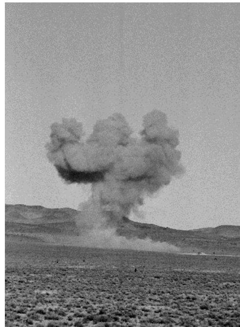
Sedan crater was formed when a 104-kt explosion buried under 635 ft of desert alluvium was fired at the NNSS on July 6, 1962, displacing 12 million tons of earth. The crater is 320 ft deep and 1,280 ft in diameter.
