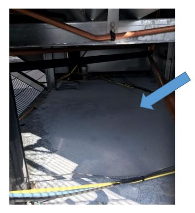
Minimizing moisture build up can help in minimizing WSS, but in most cases, it can't be avoided. WSS will not impact the service life of HVAC equipment nor will it impact the warranty of the product.
