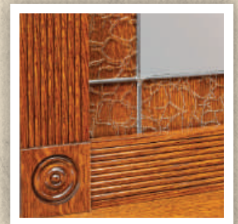
Crackled glass feature around mirror
