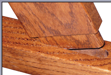
Mortise & Tenon Construction
