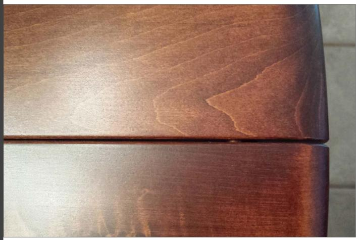
The photo above is the result of too low humidity, creating a gap at the ends of the joints. If the humidity is too high, the table will gap at the center of the joints.
