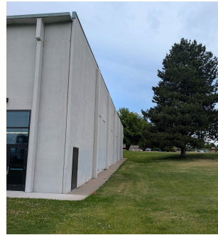
Repairs to Aquatic Center storm water drainage
