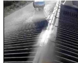
Sprinklers on the outside of roof.
