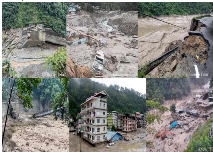
Fig. 1 Damage Caused by the Teesta Flash Floods in 23–24
