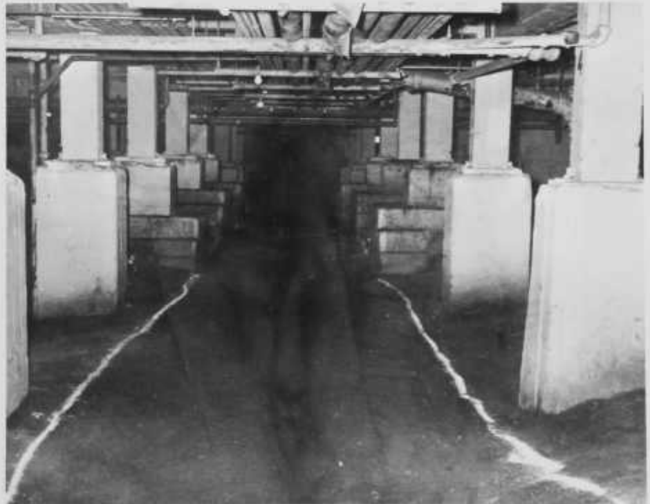
To bang my head on the pipes no more.
