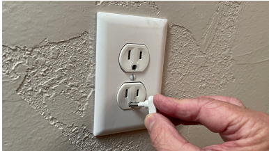
Plug white ground cord into wall
