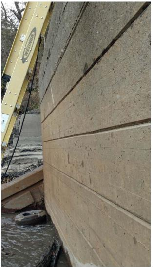
Figure 2, upstream lift joints on left spillway
