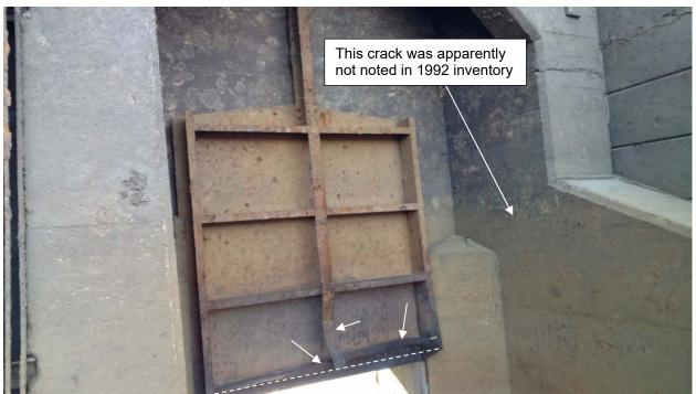
Figure 16. Looking southward at sluice gate, note damage to lower chord (log strikes) and strapping
