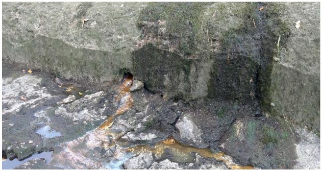
Figure 8. Typical discharge for clay tile foundation drains, possibly containing iron bacteria (red stains, labeled as "ochre" in the 1992 documents) and indicating significant levels of calcite deposits in drains (2020 minus 1966 is only 54 years, but 6" drain exits are partially blocked with calcite)
