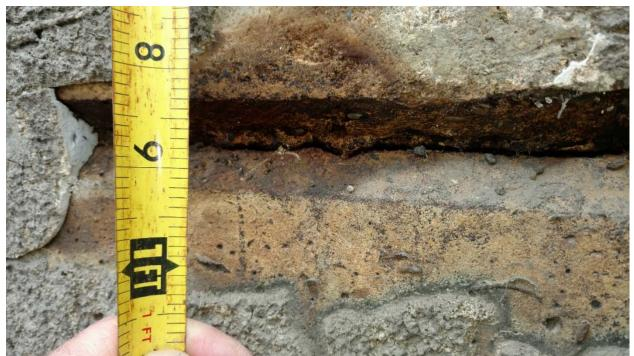
Figure 4. Closeup of coated lift joint shown on right side of Figure 3, approximate elevation 819.3
