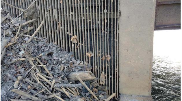
Figure 17. Trashrack, plugged 50%. Also note sand deposits faintly visible in intake bay behind trashrack. Powerhouse intake bay gate is also faintly appearing behind trashrack – note that this gate's invert sill is several feet higher than the sluiceway gate.
