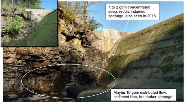
Figure 7. Downstream face of spillway near right abutment. Inset shows condition in 2015.
