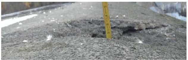
Figure 9. Looking eastward along spillway crest at spalling loss of 0.33 feet of concrete depth along deep longitudinal crack that runs from spillway crest down through at least one lift joint. Crack (but not the spall) is shown in October 1992 crack inventory, and no post-tensioned anchor is within damaged concrete area.
