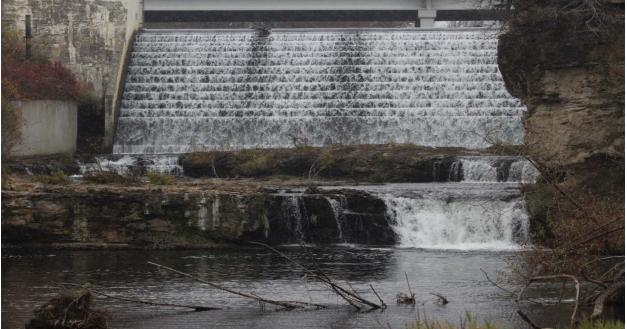
Figure 18. Looking upstream at Junction Falls tailrace. Note that waterline of scour hole is well downstream of spillway toe. However, Ayres did not walk on the toe of the Junction Falls spillway, so this view is as close as Ayres was able to safely access during the inspection.
