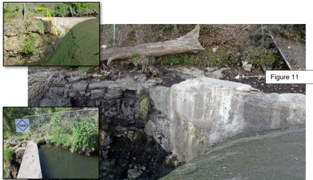
Figure 11. Looking west at right abutment, noting loss of up to 36 inches of shoreline soil. The tree trunk is approximately 21 inches in diameter at breast height for scale reference. Insets show 2015 condition.
