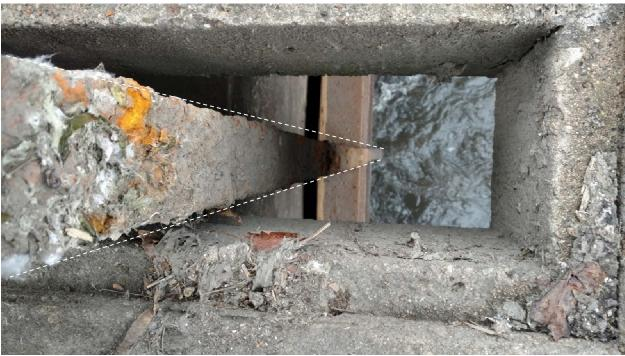
Figure 15. Looking downward at sluice gate stem, note loss of structural section, severe corrosion, and possible bow (dashed lines indicate expected edge of beam). Gate was extremely difficult to operate.
