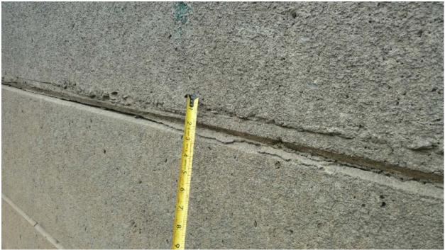
Figure 5. Separation of second lift joint, approximate elevation 817.8. Separation does not look recent.
