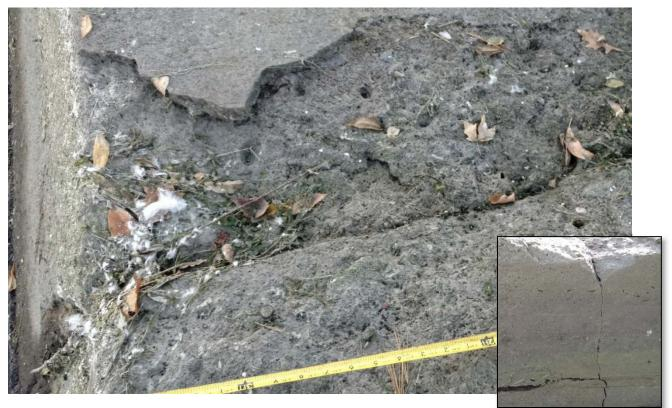
Figure 10. Another large spall, looking at top of spillway with upstream face inset to right. This crack extends through at least two lift joints, perhaps this is the same spall noted in 1992 but repaired thereafter. Inset shows view of this crack from upstream after cleaning – note how crack goes down at least through two lift joints (three horizontal monoliths).
