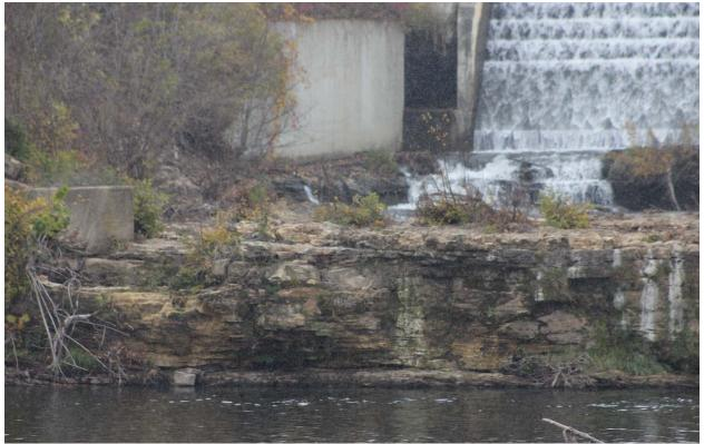
Figure 19. Looking northward at tailrace of Junction Falls. The scour hole along the training wall does not seem to be under the wall, though Ayres did not dive or hydrosurvey the ponded water.
