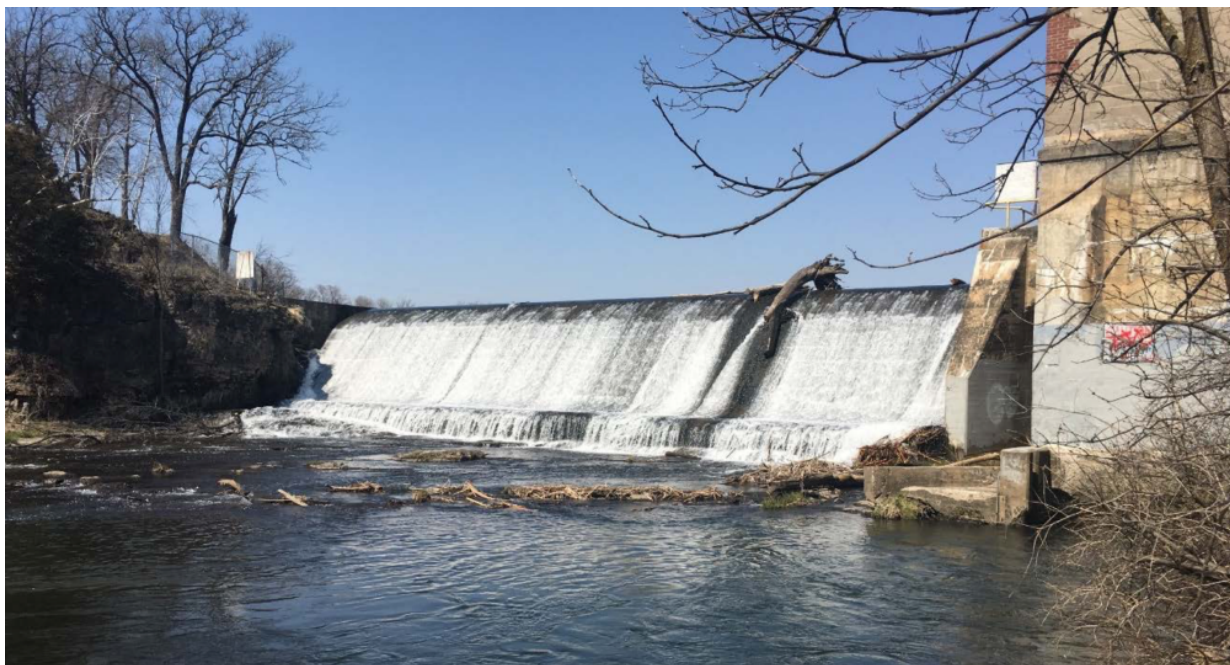
Powell Dam (Photo courtesy Kinni Corridor Project Committee)
