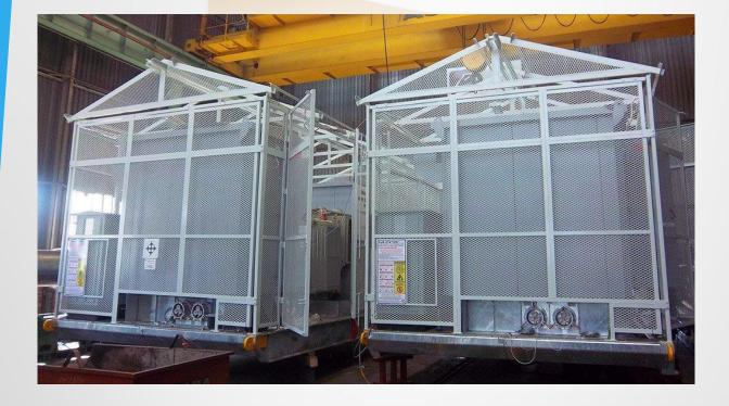
Skid Mounted Substation (SMS) which contains of RMU as per client requirement, Transformer, Low Voltage Distribution Board/Low Voltage Feeder Pillars following on a skid base. Substation includes a skid base that by default is constructed to a very robust and proven design ensuring they are capable of being towed or pushed into position in adverse conditions. The base is usually hot dipped galvanized and can be provided with towing bollards, floating axles, removable rubber wheels etc.
