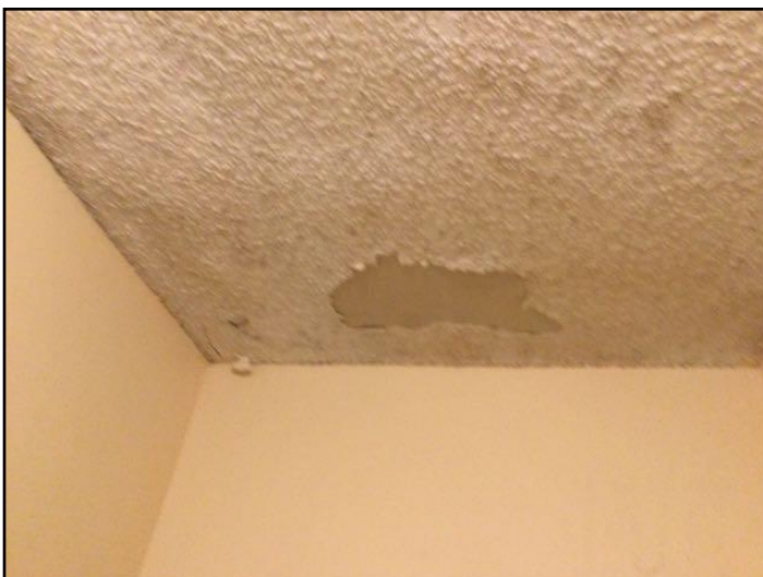
46. Water damage
