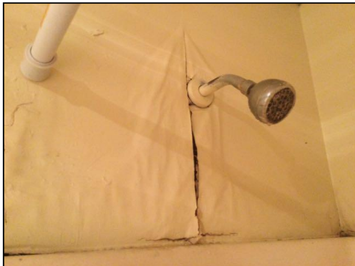
49. Water damage
