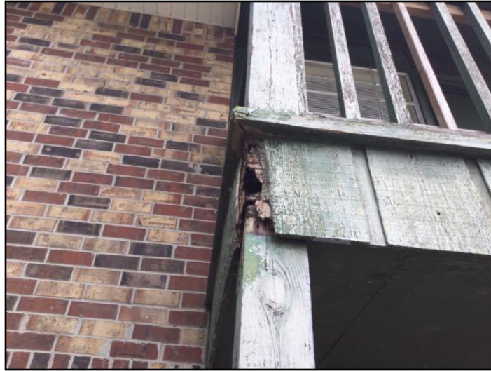
24. Rot or insect damage
