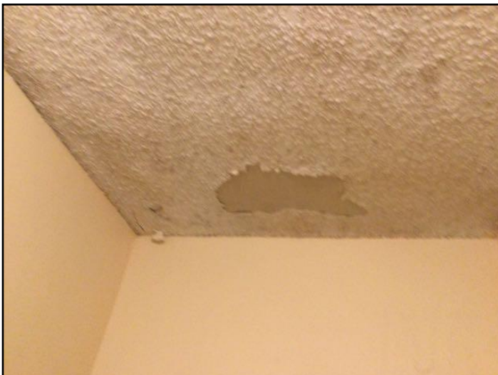
18. Water damage
