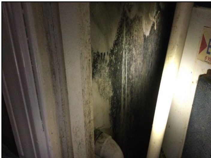
48. Water damage
