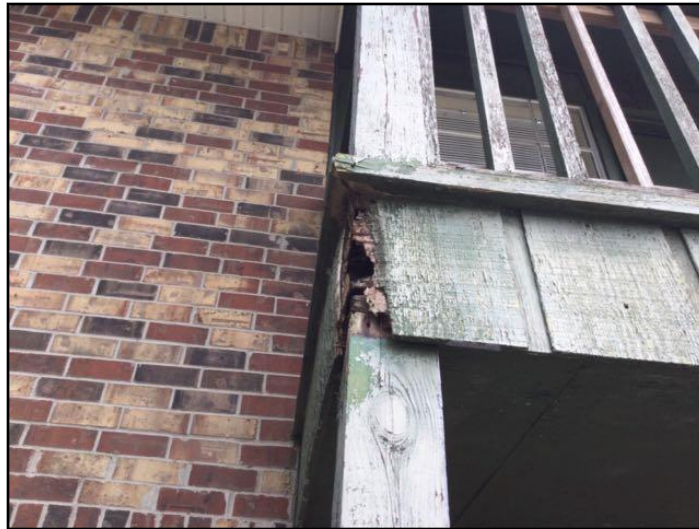
2. Rot or insect damage
