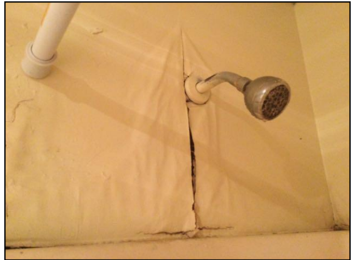
21. Water damage
