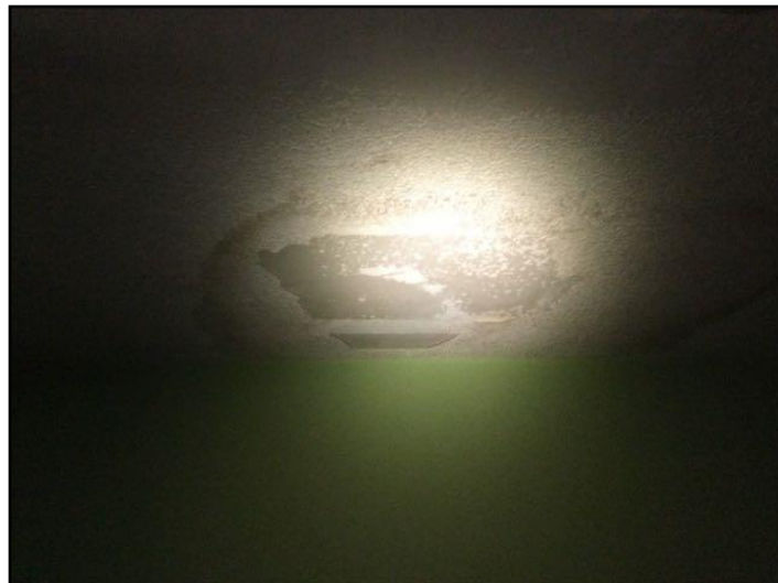
52. Water damage
