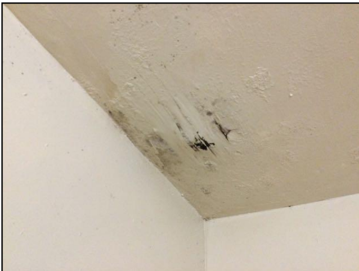
51. Water damage
