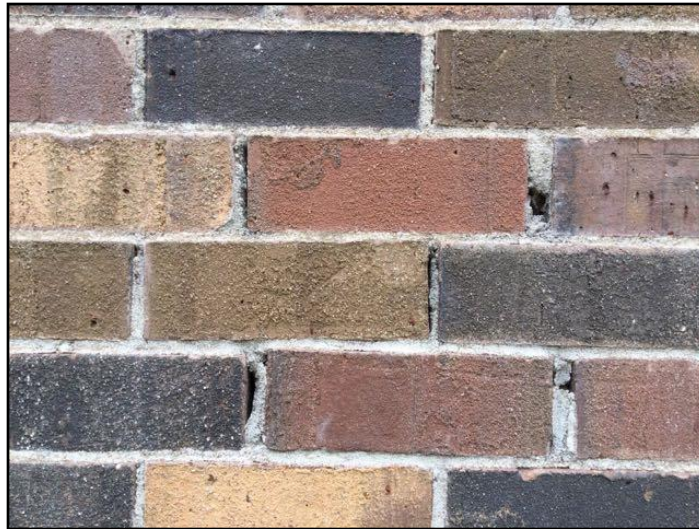
28. Masonry deterioration
