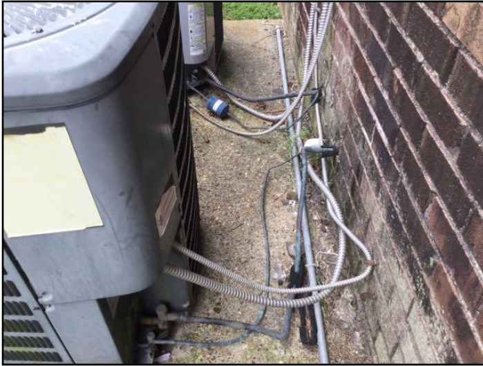
43. Insulation - missing
