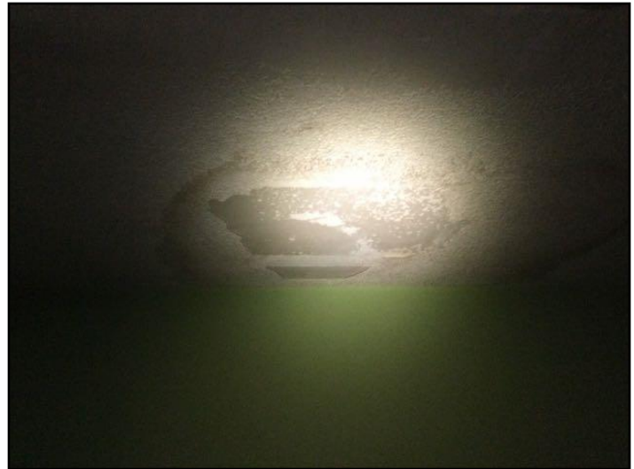
22. Water damage
