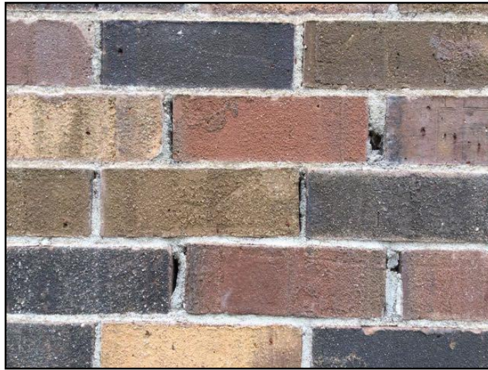
4. Masonry deterioration
