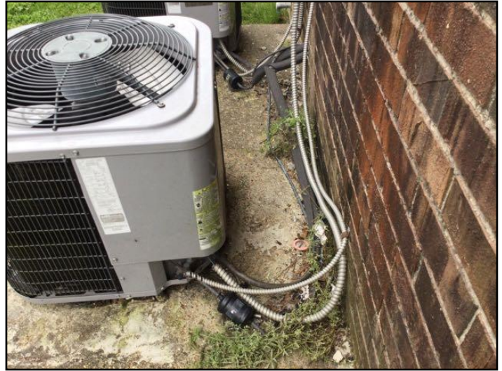
44. Insulation - missing
