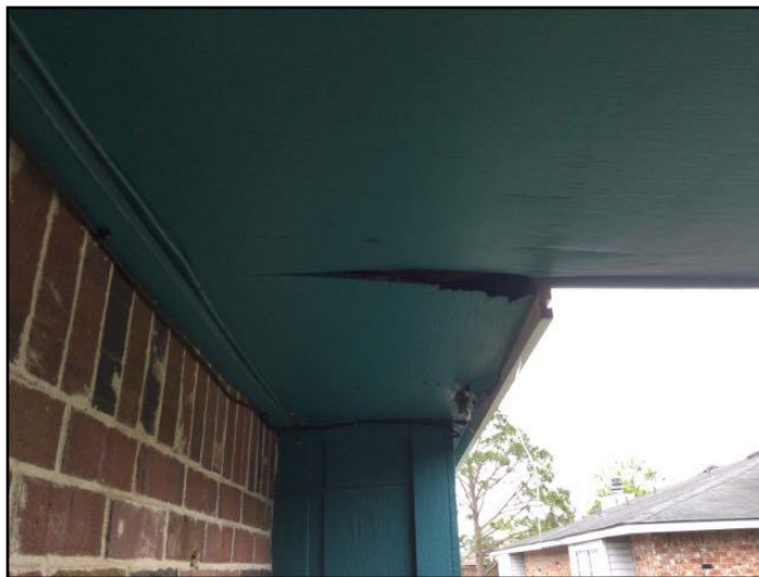
25. Rot or insect damage
