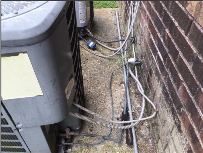
14. Insulation - missing
