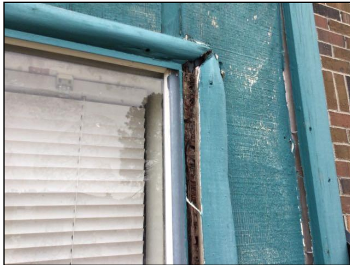
27. Rot or insect damage
