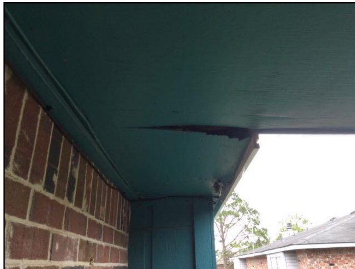
1. Rot or insect damage
