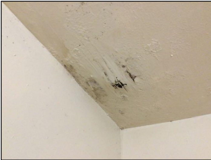
21. Water damage
