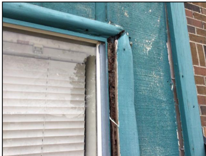
3. Rot or insect damage
