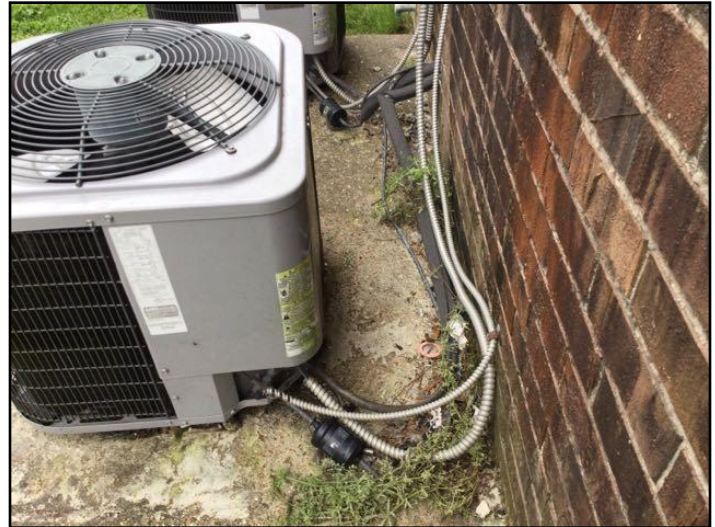
15. Insulation - missing
