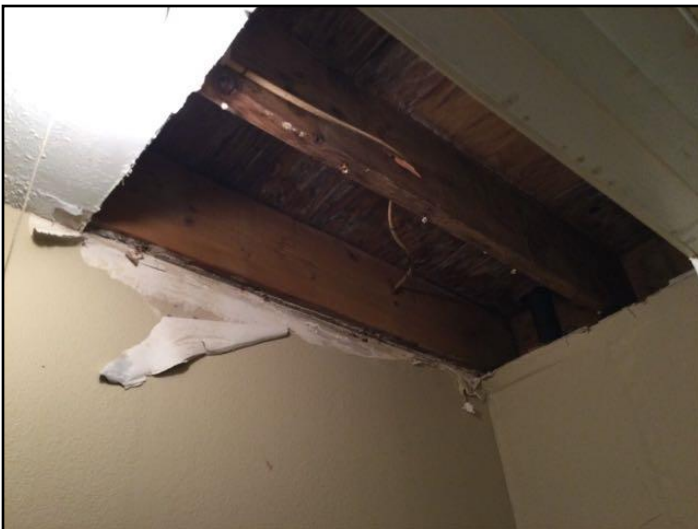
19. Water damage
