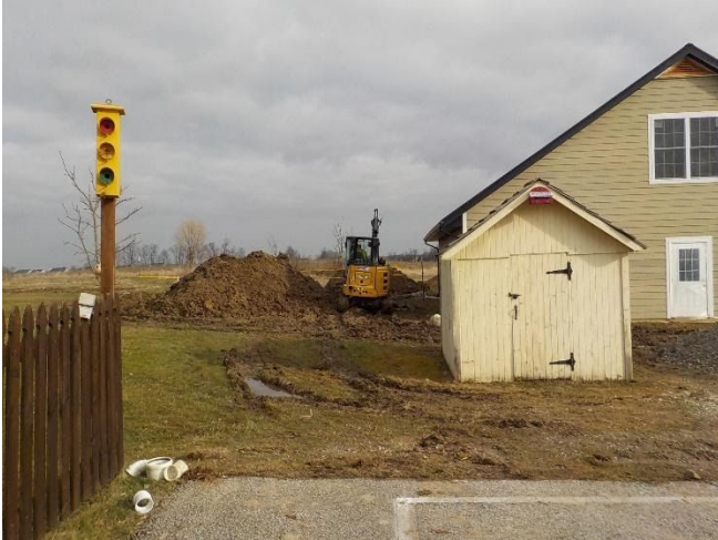
A little muddy, but work continues, west of the building
