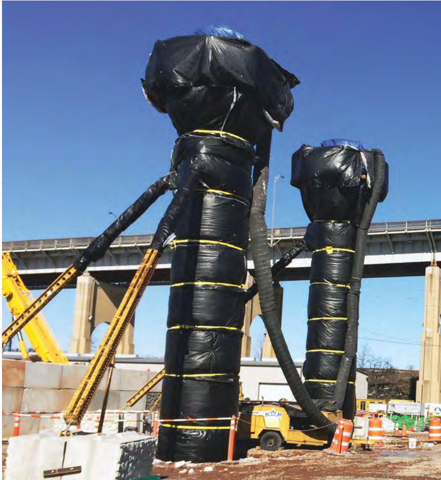
Insulated columns for a bridge project. Photo: John Gajda.
