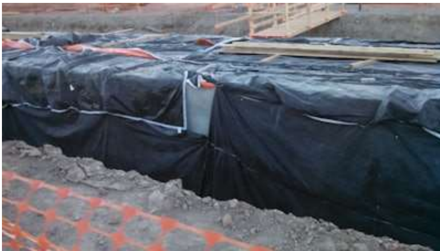
The area not insulated in the center of the photo can dissipate energy in a much wider area than the actual area of the exposure. Photo Credit: John Gajda
