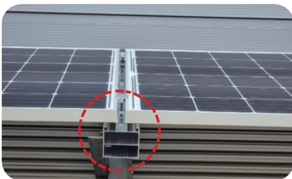
● Module integral roofstructure frame
