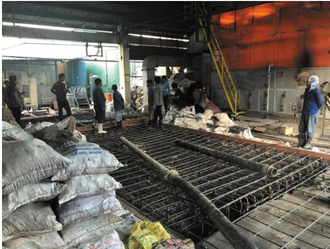
KLT Fruits Inc. First Cavite Industrial Estate, Dasmarinas Cavite 80ton Foundation for Boiler Room
