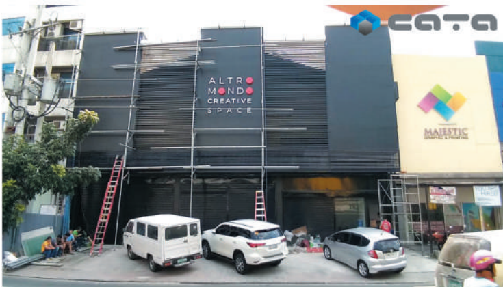
ALTRO MONDO BUILDING, MAKATI Design and Build
