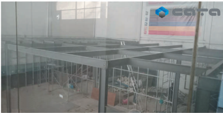
1159 Warehouse Chino Roces, Makati - Design & Build 700sqm
