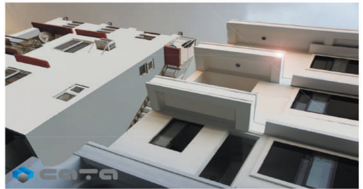
CRUZ TWIN TOWER Mandaluyong City Design & Build
