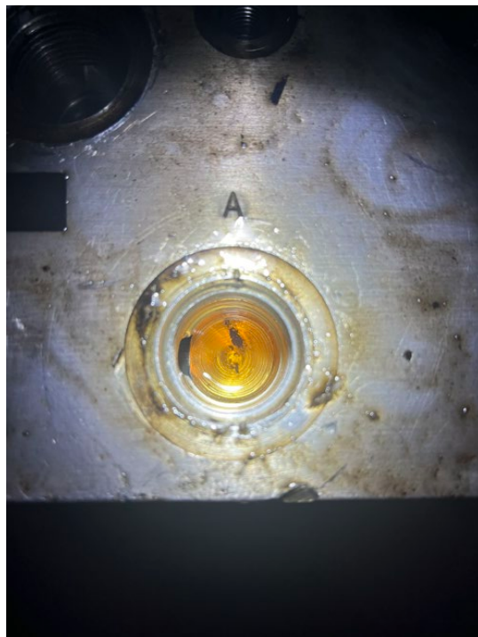
Photo 20 - Chipper Lube Oil Circulation Block Contamination
