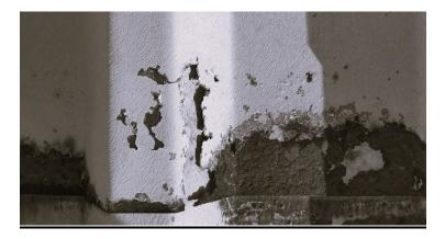
The major cause of metal roof corrosion is contact of the metal with water over long periods of time, which leads the metal to rust. This is usually caused by inadequate drainage of water from the hangar after it rains. Many of the hangars have gutter systems (including shared gutters between hangars) which have been damaged or compromised by water, wind, nesting birds and other factors, and may be inadequately sloped.
