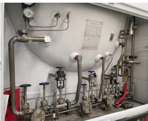
PANEL DE CONTROL
