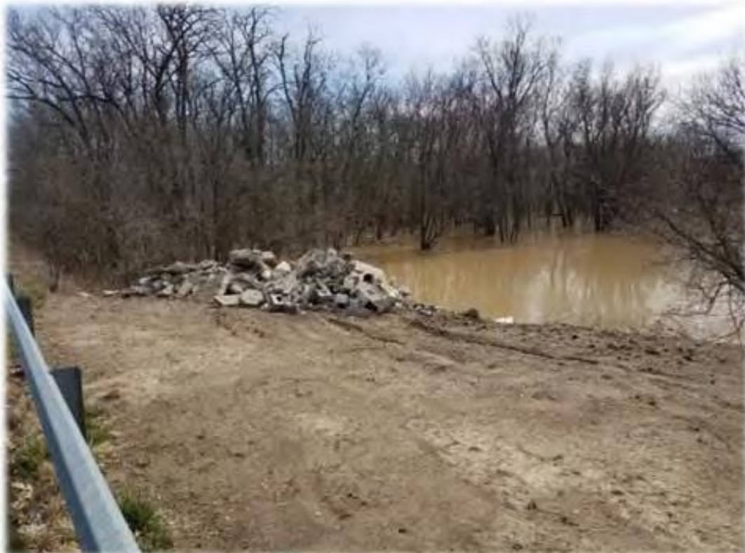
Looking southeast upstream from Road 1100S guardrail (photo courtesy Christopher Burke Engineering)
