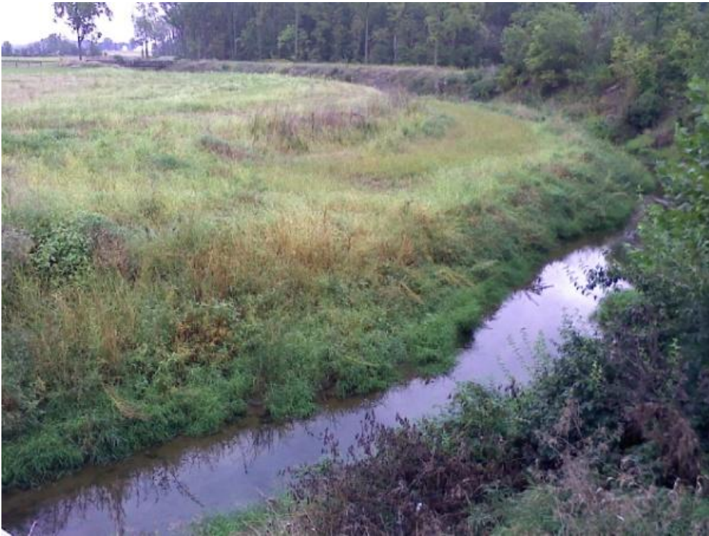
Photo 1: 2-stage Ditch on Eight Mile Creek CR 1000 N – CR 100 E (WQM site 2).
