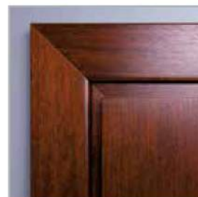
interconnection of architraves at the 45° angle
