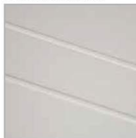
milling on the door leaf surface, 4 mm wide on versions A1-A3 and B2-B6
