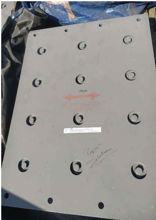
Anchored Type Elastomeric Bearing
