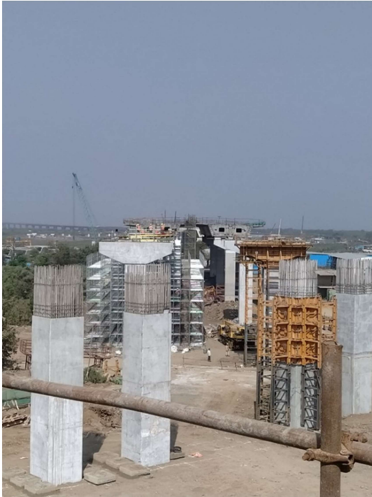
Here steel structure will be provided having the main span as 60m
