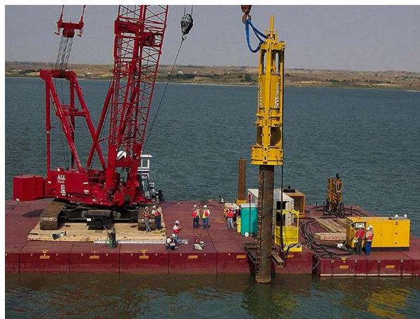
Barge and Pile Driver
