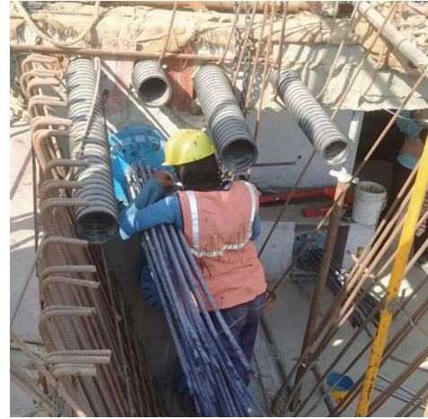
Set-up for Prestressing
