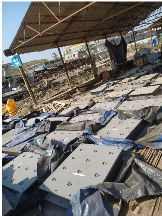
Anchored Type Elastomeric Bearing
