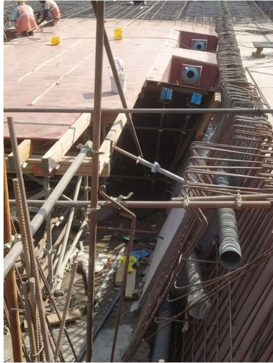
Sheathing pipe placed in for prestressing
