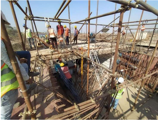
Set-up for Prestressing
