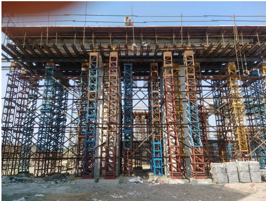
Supports provided for cast-in-situ pier cap near railways tracks (span 60m)
