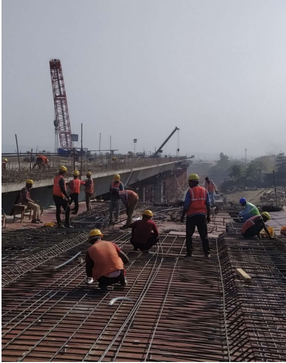
Cast-in-situ span
