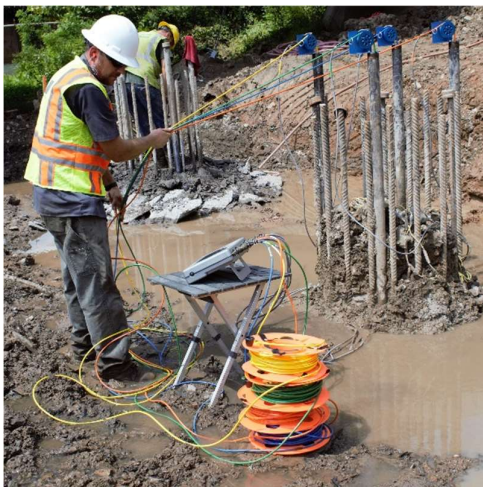
Ultrasonic Cross-Hole Testing on Pile
