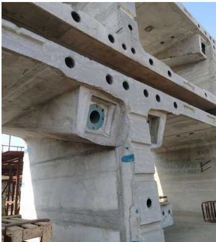
Cantilever tendons Anchor Blister
