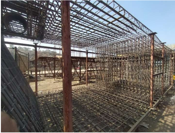
Reinforcement Cage of the segment in the casting yard
