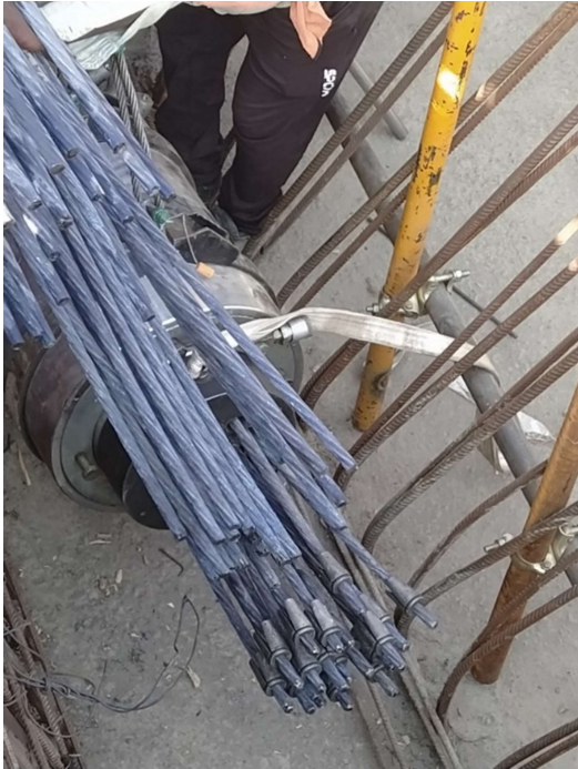
Wedges passed through the tendons
