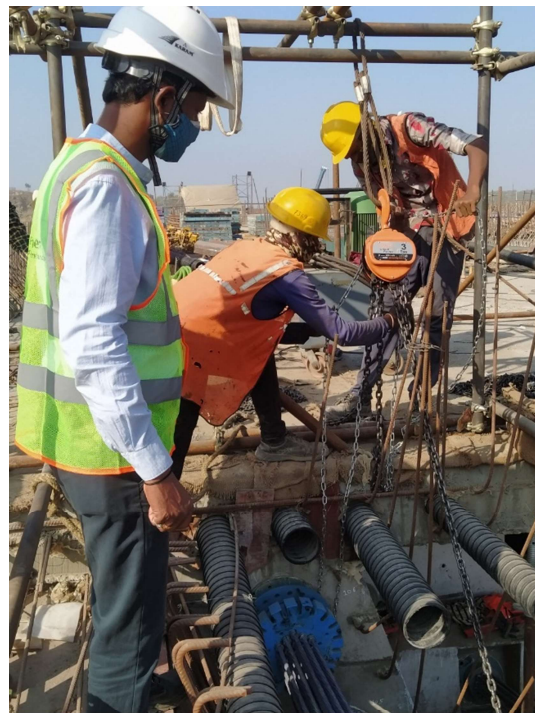
Chain pulley used for the adjustment of the jack
