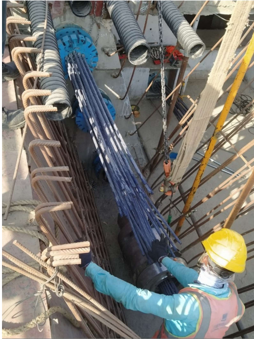
Tendons passed through jack for stressing process
