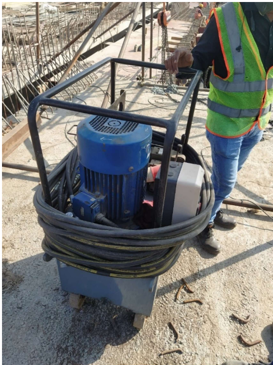
Pressure pump for applying pressure to tendons
