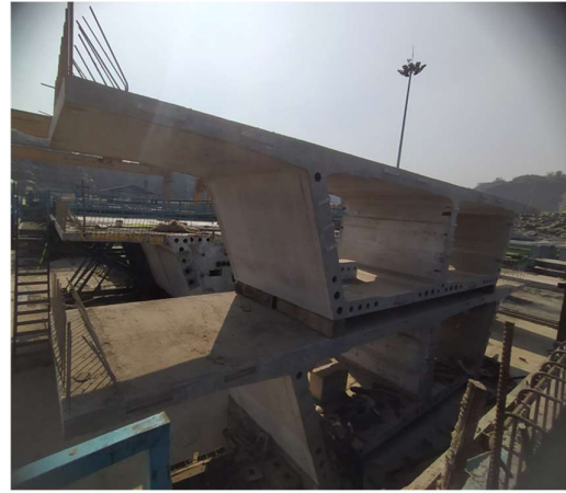
Segment after casting
