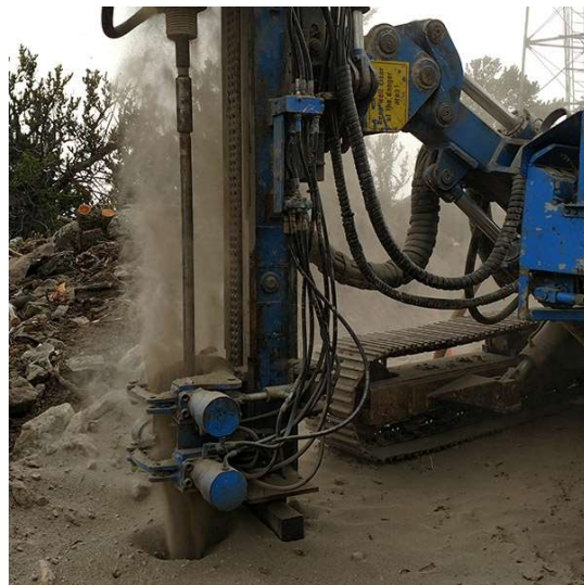
Drilling of Rock Anchor
