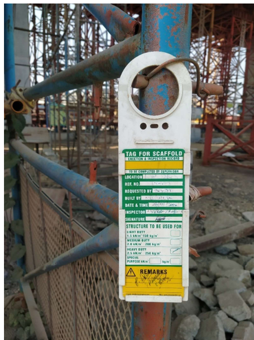
Tag provided at the entrance of staircase
