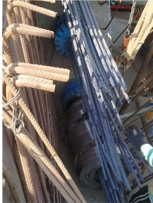
Tendons passed through jack for stressing process
