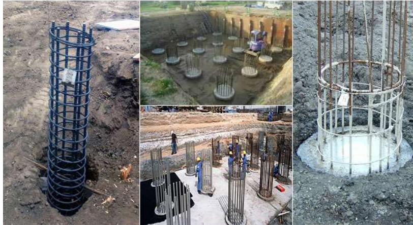
Bored cast-in-situ Pile
