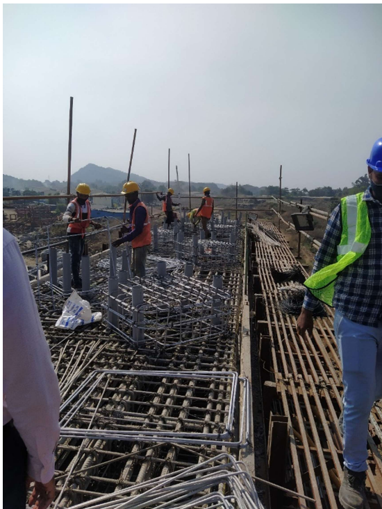
Pedestal provided on Pier cap
