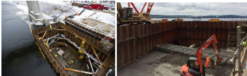
Creating Dry work space by pumping the water out
