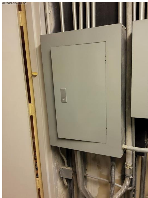
Photo # 50. Item 7.19.a. Level 20. Meter Room. Panelboard 20H. Missing panel Identification.
