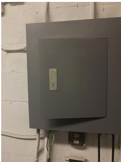
Photo # 69. Item 7.30.a. Level Roof. Mechanical Room. Panelboard REL. Missing panel Identification.
