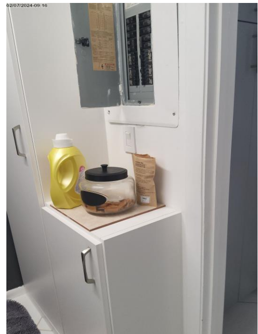
Photo # 116. Item 28.6. Electrical panel: working space clearance violation.
