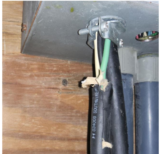
Photo # 26. Item 7.8.c. Level 1. Main Electrical Room. Panel NO ID. Connector cable to panel is detached.
