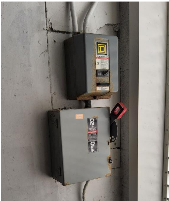
Photo # 73. Item 12.b. Roof. Enclosed Circuit breaker not marked to identify the load.
