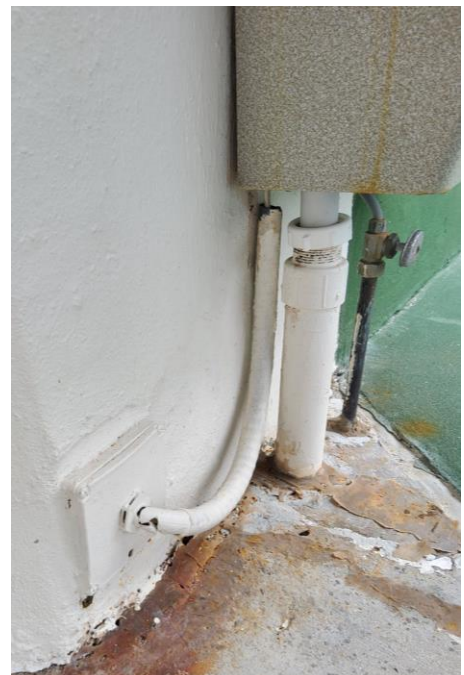
Photo # 88. Item 17.m. Drinking fountain. Flexible detached and broken connector.
