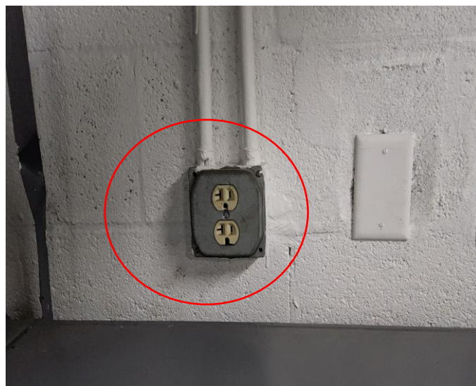
Photo # 80. Item 17.f. Level 2. Roof. Mechanical Room. Missing GFCI protection for receptacles.
