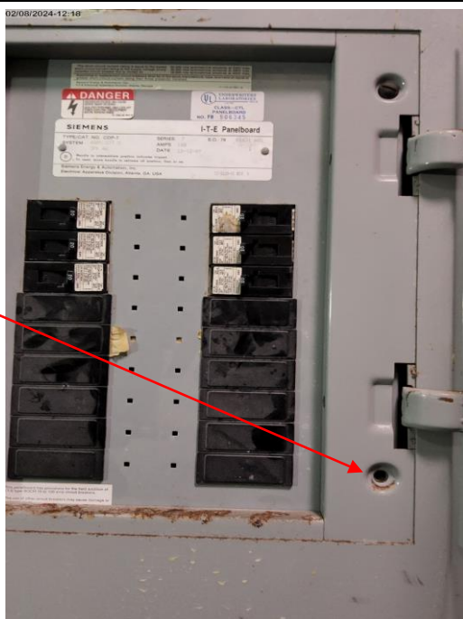
Photo # 19. Item 7.5.b. Level 1. Main Electrical Room. Panel EH. Missing screws.
