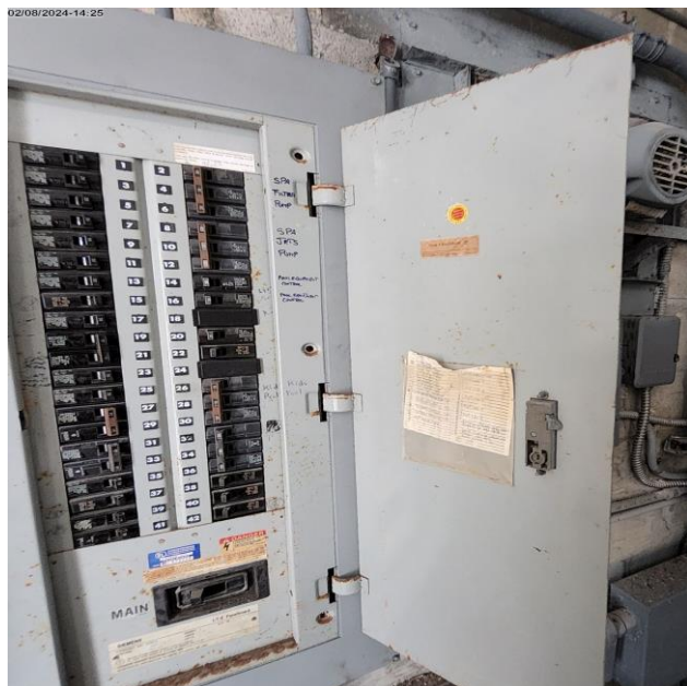
Photo # 37. Item 7.12.b. Pool. Electrical Room. Panel NO ID. Missing proper circuit identification.
