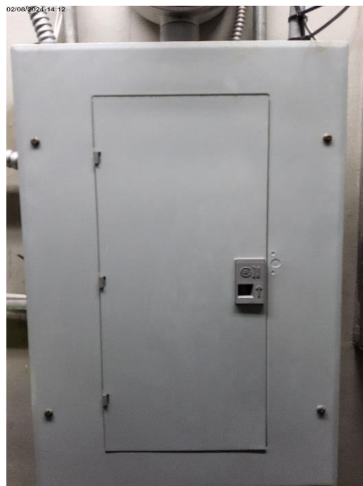
Photo # 46. Item 7.17.a. Generator Room. Panel No ID. Missing panel Identification.
