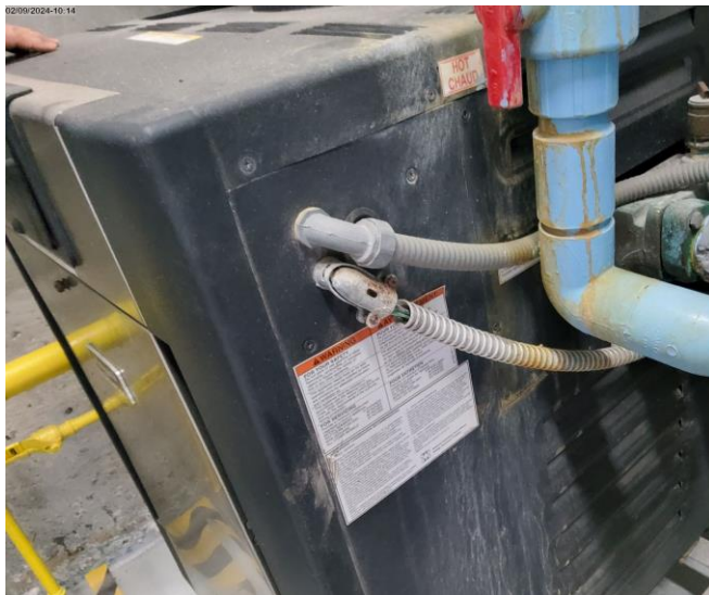
Photo # 89. Item 17.n. Water heater. Flexible detached and broken connector.
