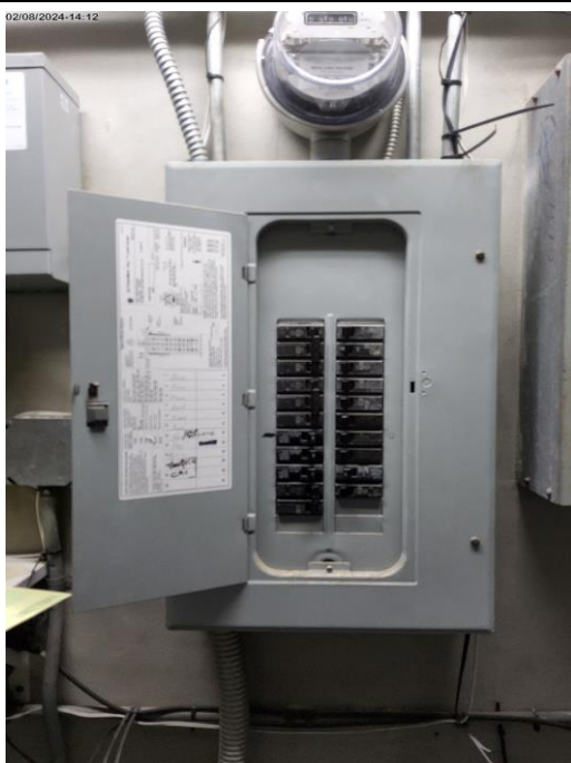
Photo # 47. Item 7.17.b. Generator Room. Panel No ID. Missing proper circuit identification.
