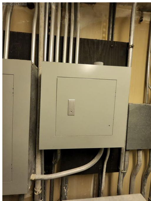
Photo # 52. Item 7.20.a. Level 20. Meter Room. Panelboard 20EH. Missing panel Identification.
