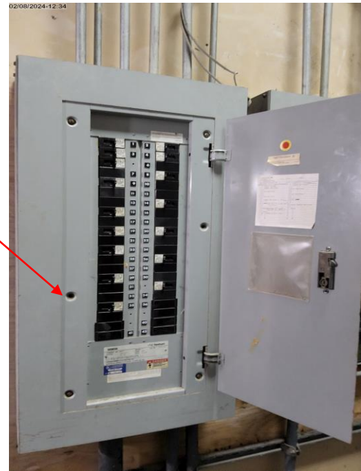
Photo # 34. Item 7.11.c. Level 1. Main Electrical Room. Panel NH. Missing Screws.
