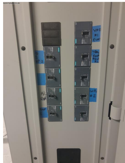
Photo # 68. Item 7.29.b. Level Roof. Mechanical Room. Panelboard No ID. Missing proper circuit identification.
