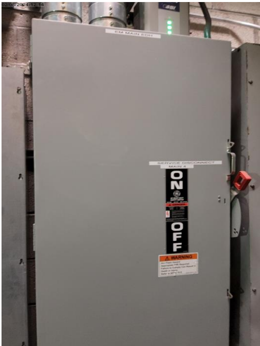
Photo # 3. Item 3.3. Electrical Room. EM Main #4. Disconnect Switch. All service equipment must be identified
