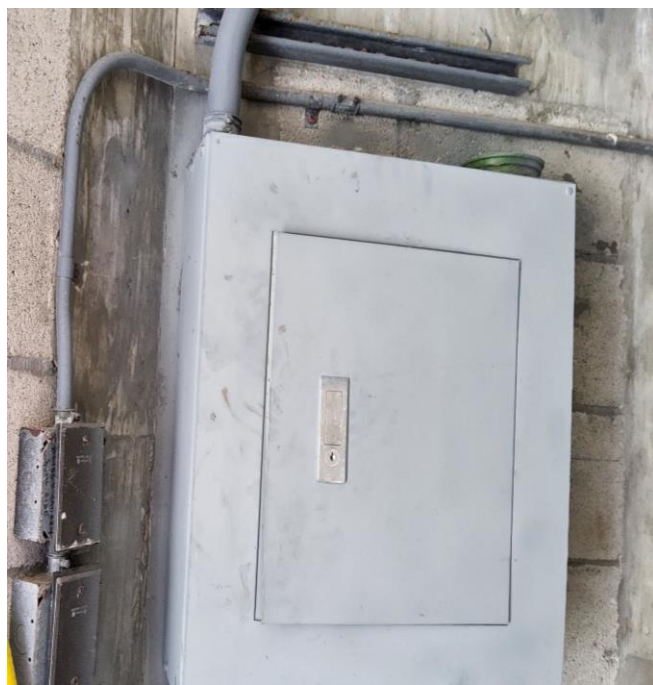
Photo # 43. Item 7.15.a. Pool. Electrical Room. Panel NO ID. Missing panel identification.
