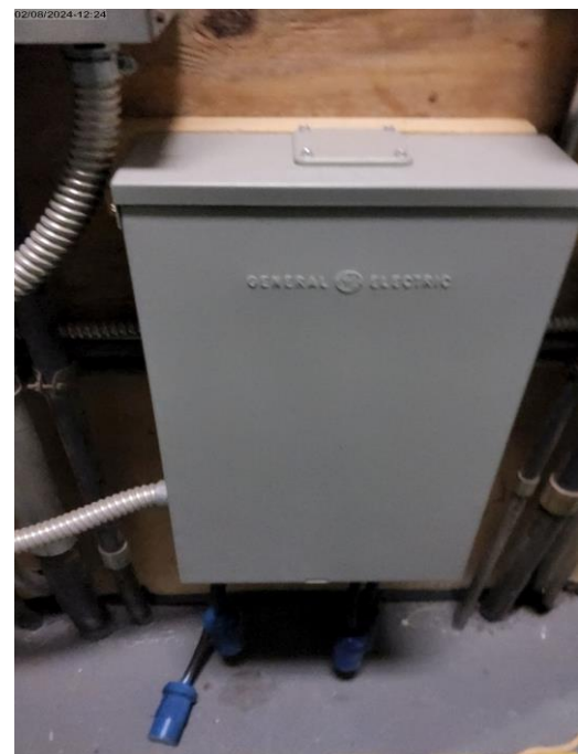
Photo # 24. Item 7.8.a. Panel NO ID. Main Electrical Room. Missing panel Identification.
