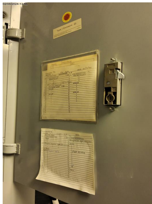
Photo # 60. Item 7.25. Level 7. Meter Room. Panelboard 7L. Missing proper circuit identification.
