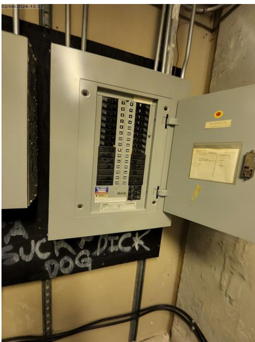
Photo # 55. Item 7.21.b. Level 20. Meter Room. Panelboard 20L. Missing proper circuit identification and missing screws.
