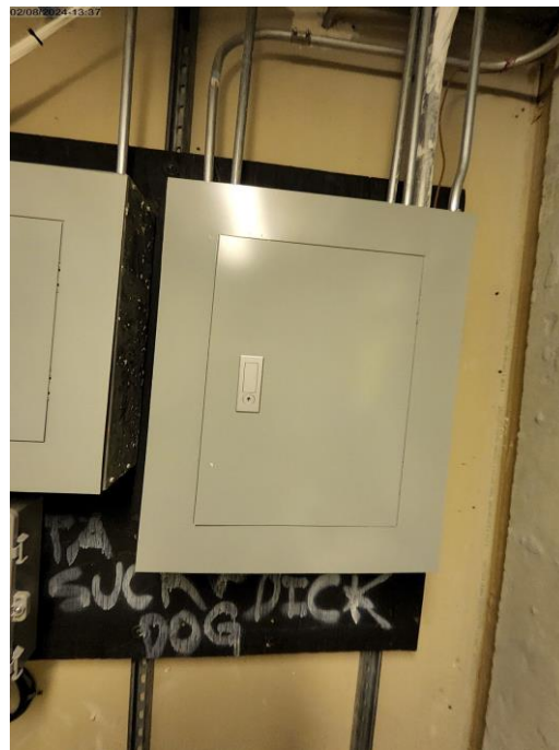
Photo # 54. Item 7.21.a. Level 20. Meter Room. Panelboard 20L. Missing panel Identification.
