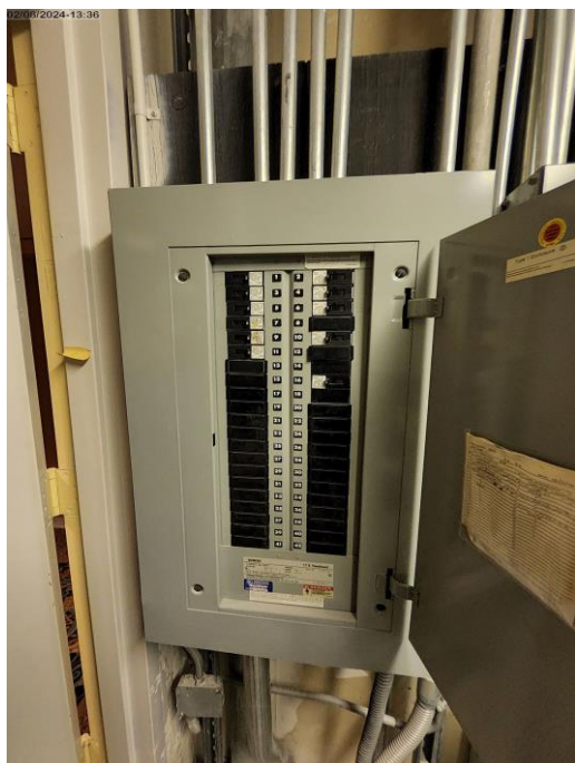
Photo # 51. Item 7.19.b. Level 20. Meter Room. Panelboard 20H. Missing proper circuit identification and missing screws.
