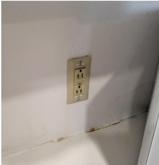
Photo # 85. Item 17.j. Club Room. Kitchen. Missing GFCI protection for receptacles - test fail.
