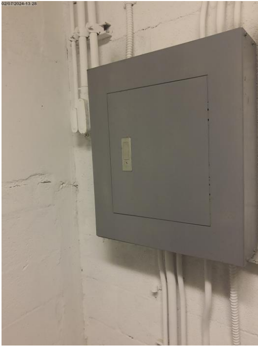
Photo # 13. Item 7.1.a. Level Roof. Mechanical Room. Panelboard No ID. Missing panel Identification.
