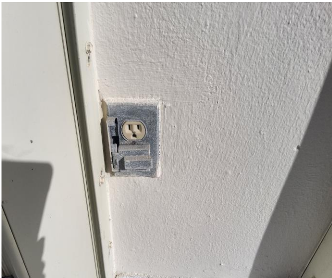
Photo # 111. Item 28.3. Missing GFCI protection for receptacles in the balcony.
