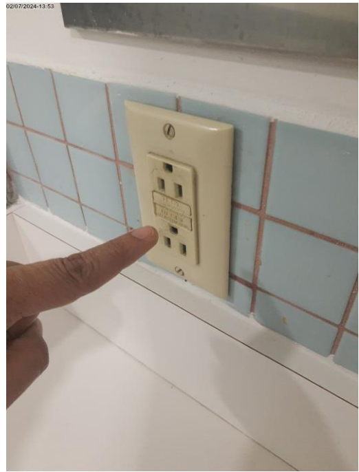
Photo # 82. Item 17.h. Restroom. Missing GFCI protection for receptacles- test fail.
