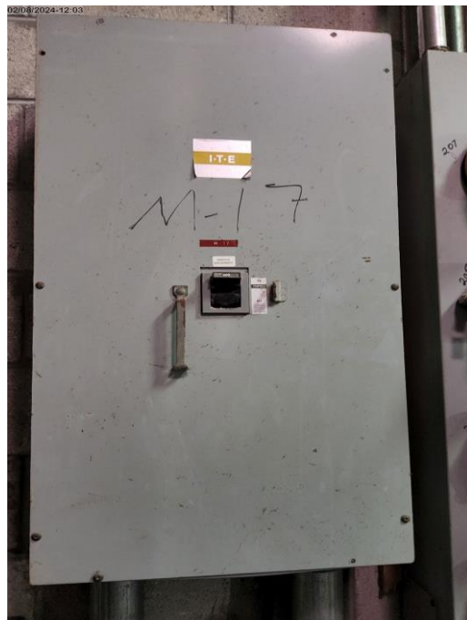
Photo # 74. Item 12.c. Level 1. Main Electrical Room. Enclosed disconnect switch M17 not marked to identify the load and missing screws.
