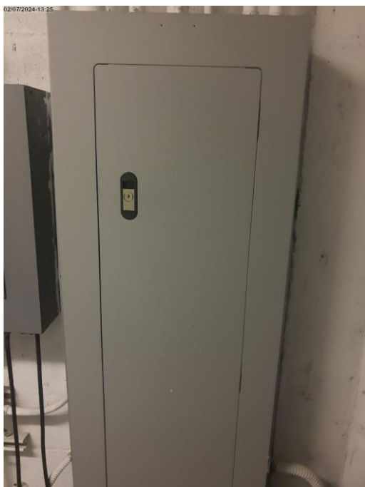
Photo # 67. Item 7.29.a. Level Roof. Mechanical Room. Panelboard No ID. Missing panel Identification.
