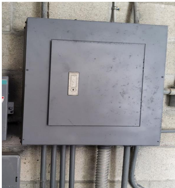
Photo # 39. Item 7.13.a. Pool. Electrical Room. Panel NO ID. Missing panel Identification.
