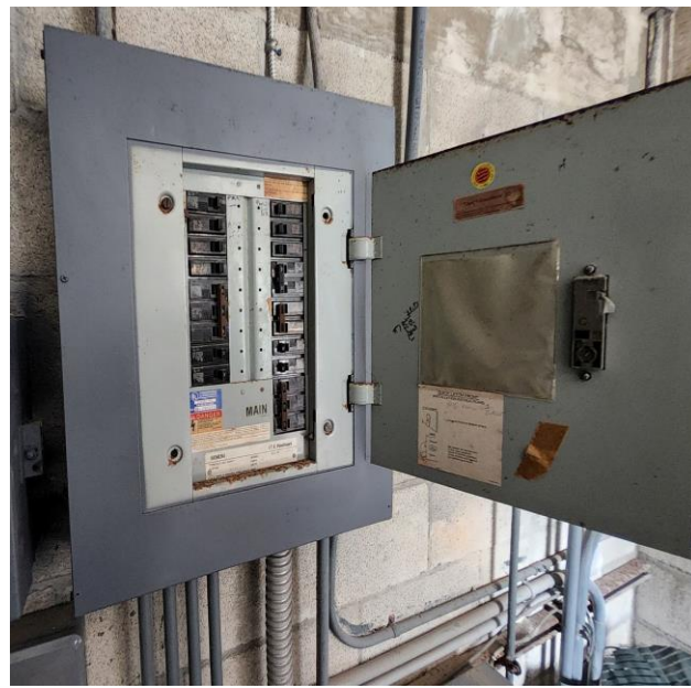
Photo # 40. Item 7.13.b. Pool. Electrical Room. Panel NO ID. Missing proper circuit identification, and missing screws.
