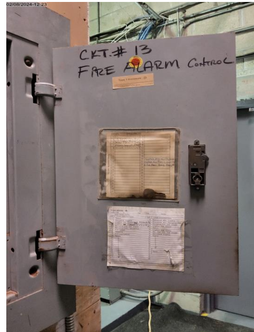
Photo # 22. Item 7.7.a. Level 1. Main Electrical Room. Panel EL. Missing proper circuit identification.
