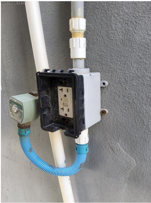
Photo # 81. Item 17.g. Roof. Missing cover weatherproof for receptacle box.
