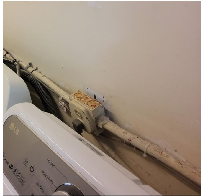
Photo # 86. Item 17.k. Laundry Room. Missing GFCI protection for receptacles.
