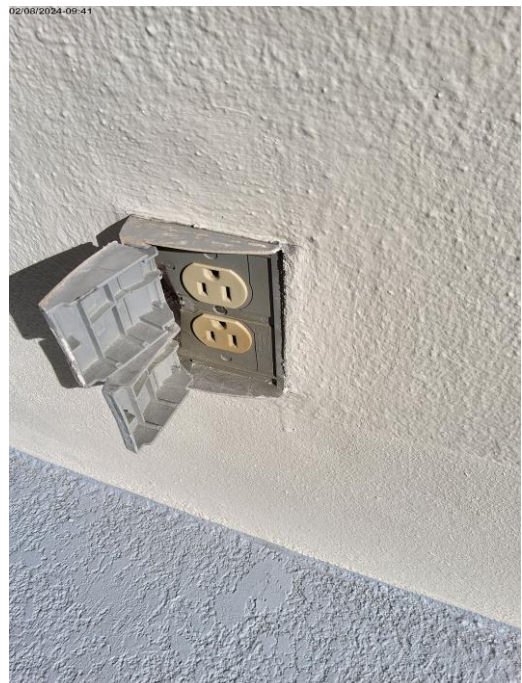
Photo # 112. Item 28.3 Missing GFCI protection for receptacles in the balcony.
