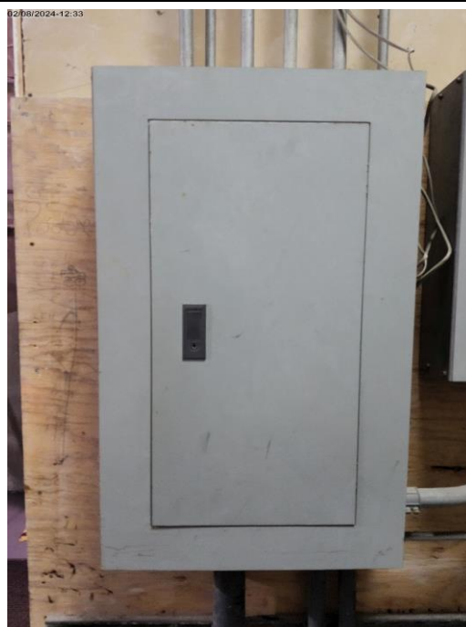
Photo # 32. Item 7.11.a. Panel NH. Main Electrical Room. Missing panel Identification.
