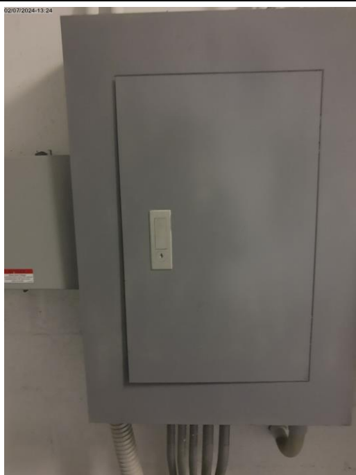
Photo # 63. Item 7.28.a. Level Roof. Mechanical Room. Panelboard RL. Missing panel Identification.
