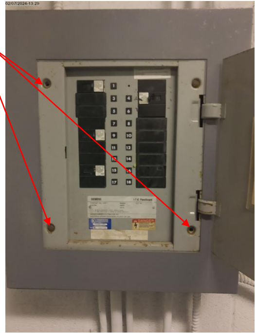
Photo # 14. Item 7.1.b. Level Roof. Mechanical Room. Panelboard No ID. Missing screws.
