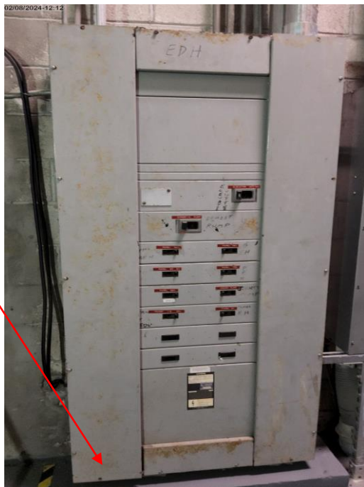
Photo # 17. Item 7.4. Level 1. Main Electrical Room. Panel EDH. Missing screws.
