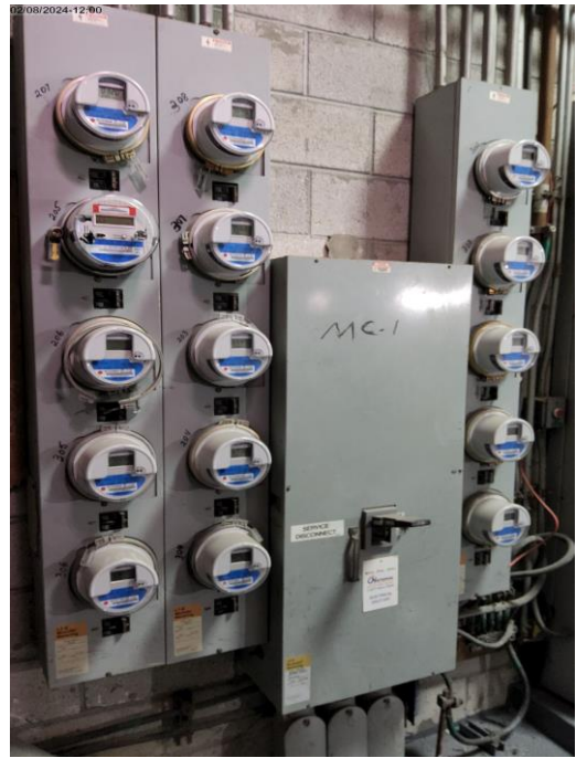
Photo # 2. Item 3.2. Electrical Room. MC-1. Disconnect Switch. All service equipment must be identified.
