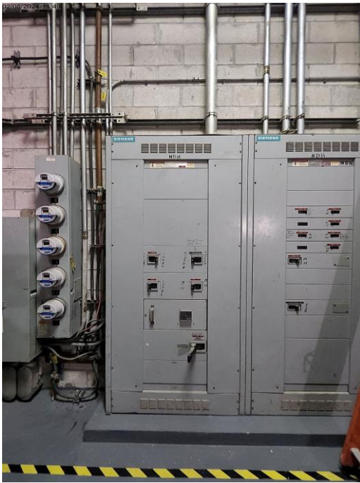
Photo # 1. Item 3.1. Electrical Room. NDH. Missing proper panel Identification - X of Y. All service equipment must be identified
