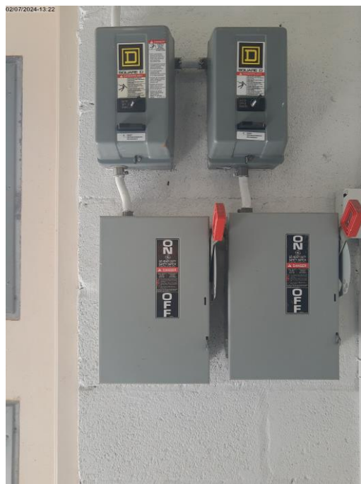
Photo # 72. Item 12.a. Roof. Enclosed Circuit breaker not marked to identify the load.
