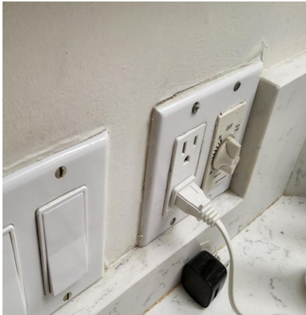
Photo # 109. Item 28.2. Missing GFCI protection for receptacles in the bathroom.
