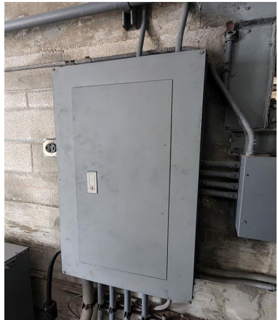
Photo # 36. Item 7.12.a. Pool. Electrical Room. Panel NO ID. Missing panel Identification.
