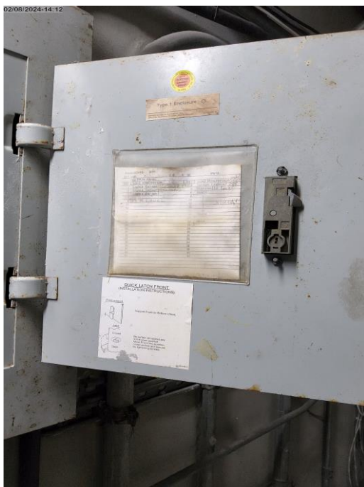
Photo # 45. Item 7.16. Generator Room. Panel 3. Missing proper circuit identification.
