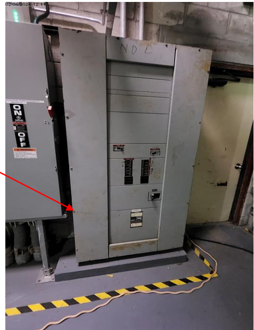
Photo # 16. Item 7.3. Level 1. Main Electrical Room. Panel NDL. Missing screws.
