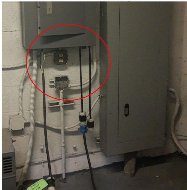
Photo # 77. Item 17.c. Roof. Electrical Room. Missing Cover for Junction Box and missing GFCI protection for receptacle
