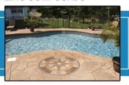
Deco Guard Plus is a non yellowing, high gloss, siloxane modified methyl methacrylate with excellent adhesion to properly prepared old or new concrete substrates. It's unique chemical reactive formula provides superior resistance to de-icing road salts, salt water pool systems, rain, sleet and snow compared to standard sealers used to protect exterior concrete.
