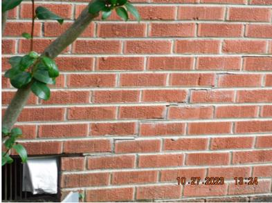
**🔧 (ED-4) Review:** Masonry siding mortar joints missing or damaged in numerous locations.
