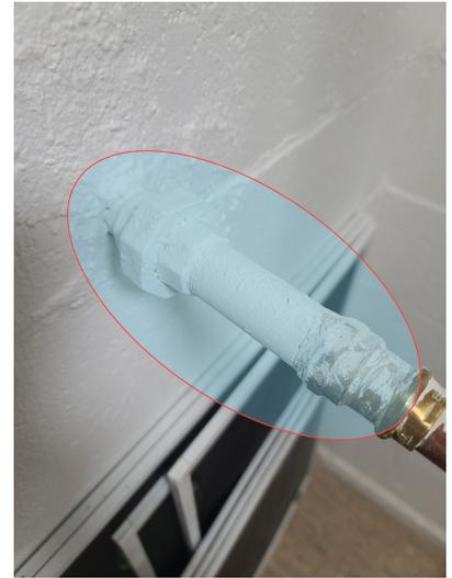
*It looks as though the main water pipe to the house is older galvanized steel.*
