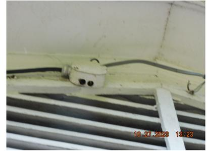
🔧 (EDFW-2) Review: Nonmetallic sheathed cable installed on the exterior of the buildings. Refer to line 5440 of the Uniform Building Inspection Report Binder.
