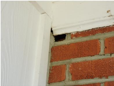
**🔧 (ED-6) Review:** Siding and roof trims appear damaged in various locations. Refer to line 1310 of the Uniform Building Inspection Report Binder.
