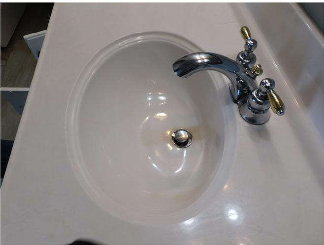
Sink missing overflows drains in sinks.
