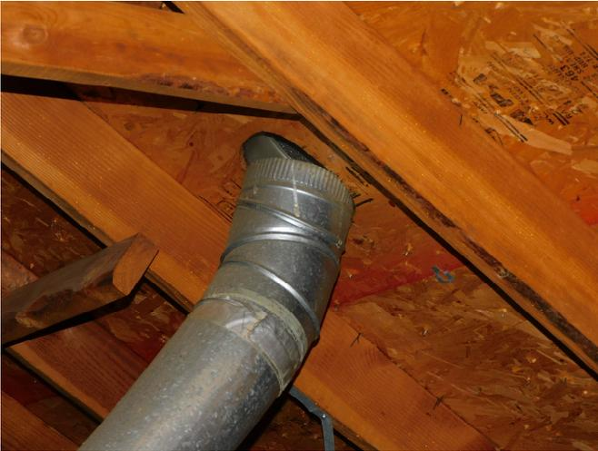
Exhaust vent not properly installed through roof.
