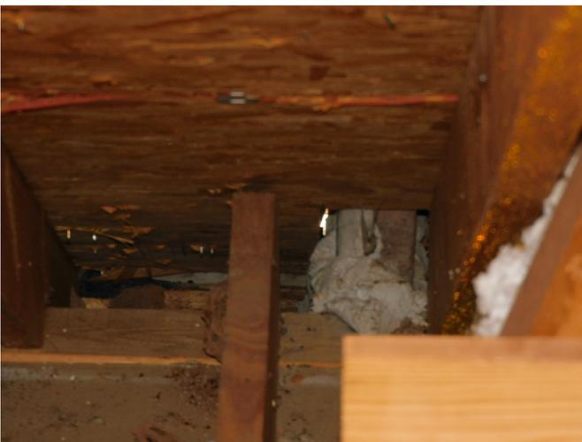
Roof decking questionable and faulty. Daylight visible through materials which if light is entering so can water.
