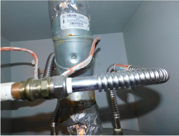
Electrical power line in contact with WH exhaust pipe.
