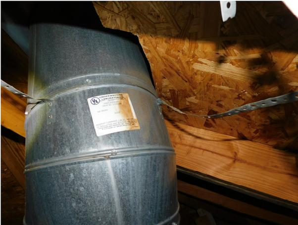
Chimney clearances through the roof improper and signs of water draining down the metal chimney.
