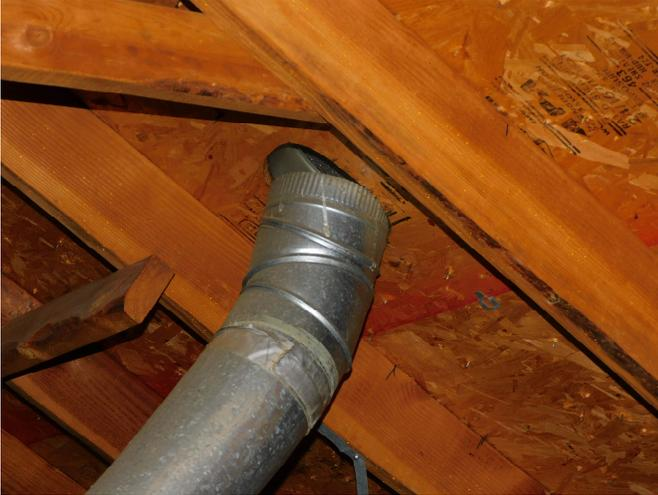
Exhaust vent not properly installed through roof.
