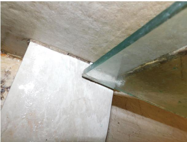
Shower grout damage and cracked. The damage grout can be leading to moisture damage in the home.
