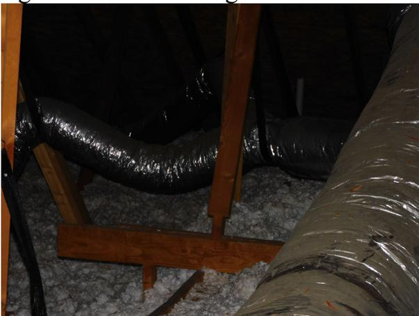
Flex ducting improperly hung or supported. This can lead to air flow issues in the home and moisture build up.
