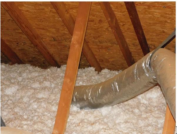
Insulation baffles missing at soffits which will lead to poor air flow and increase moisture issues.
