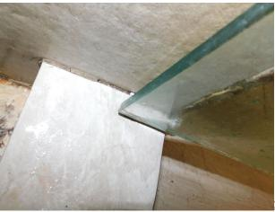
Shower grout damage and cracked. The damage grout
