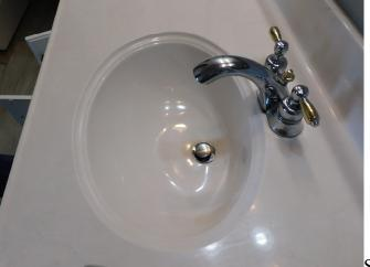
Sink missing overflows drains in sinks.
