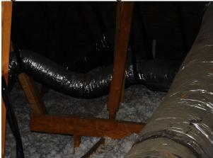
Flex ducting improperly hung or supported. This can
