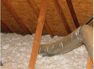
Insulation baffles missing at soffits which will lead to
