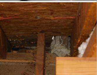
Roof decking questionable and faulty. Daylight
