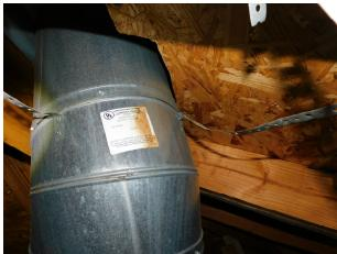
Chimney clearances through the roof improper and
