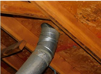
Exhaust vent not properly installed through roof.
