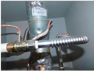
Electrical power line in contact with WH exhaust
