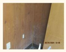
**(I-7) Review:** Visible signs of roof leakage and damage.
