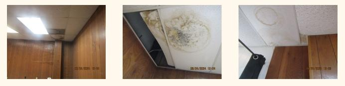
**(I-6) Review:** Wood paneling showing signs of possible water damaged and suspected mold.
