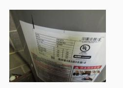
System Type: Tank Size: 50 gal Age: 2021 Energy Source: Electricity Temperature Pressure Relief Value: Inadequate Discharge - General Note
