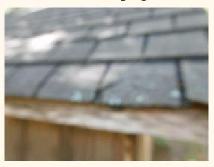
**(RCG2-1) Recommended Preventive Maintenance:** Shingles lifted which may allow wind to tear off shingles.
