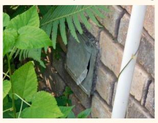
**(LF-3) Recommended Preventive Maintenance:** The dryer exhaust ductwork is dirty and needs to be cleaned for improved safety. This is important regular maintenance to eliminate a potential fire hazard.
