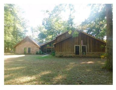
Board and batten siding home. The wood siding is cracking and gaped in numerous locations.
