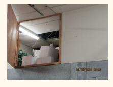
(I-9) Review: Ceiling tiles sagging and damaged. Repair of damage tiles \$500 to \$1000
