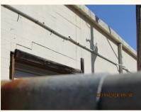
**(ED-6) Review:** Siding appears to be water damaged. Repairs for water damage \$5000 to \$1000.00
