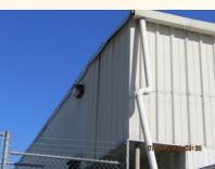
(RCG-7) Review: Gutters appear to leak. Repairs to gutter \$ 8 to 10,000
