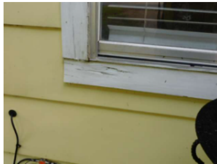
Image 1.4.2 window trim damaged
