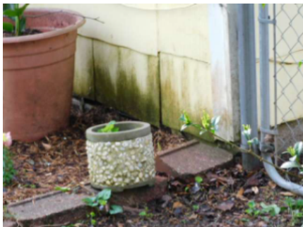
Image 1.4.4 Siding stained/damaged in contact with earth
