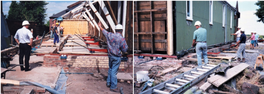
The 'Iron Church' being moved 3 metres sideways in 1995
